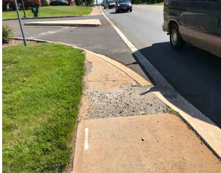
Sidewalk deterioration along Finderne Ave (left) and Union Ave (right) reduces accessibility.
