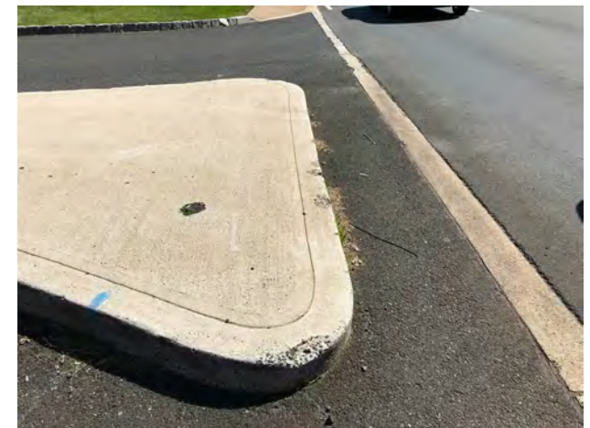
A concrete island at a parking lot entrance along Finderne Ave is not wheelchair accessible, forcing pedestrians into the high-speed roadway.
