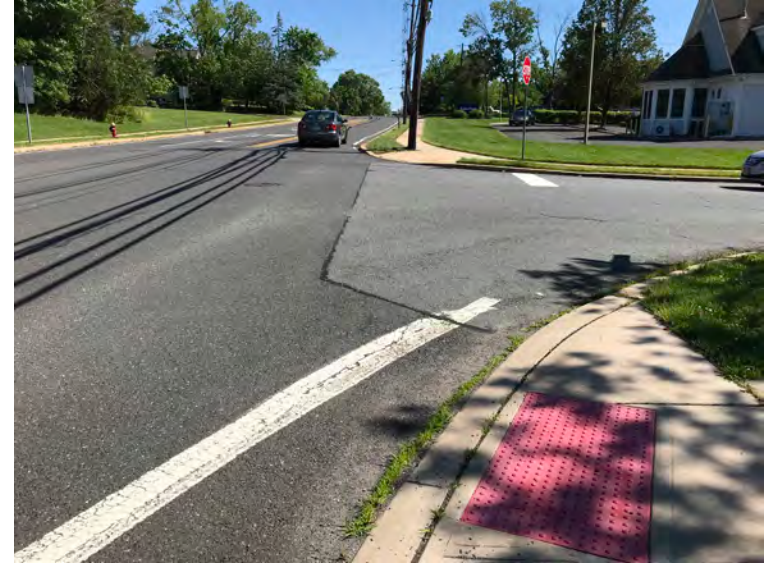
Raised sidewalk warning pad at the intersection of North Bridge Street and 7th Avenue is not aligned with the crossing, instead pointing pedestrians into the busy roadway and potentially endangering the sight-impaired (right)
