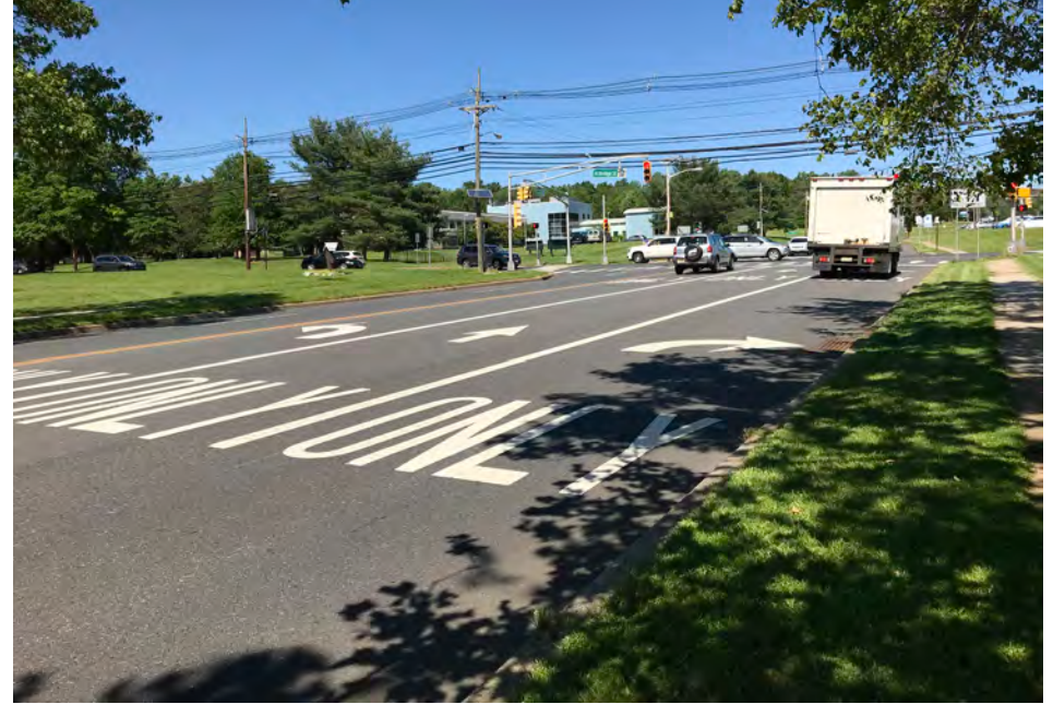
Five lanes of travel on Prince Rodgers Ave at its intersection with North Bridge St, resulting in a 70-foot crosswalk (above)
