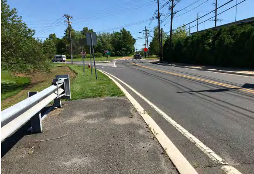
The sidewalk on the east side of North Bridge Street ends abruptly and without a marked crosswalk (left)
