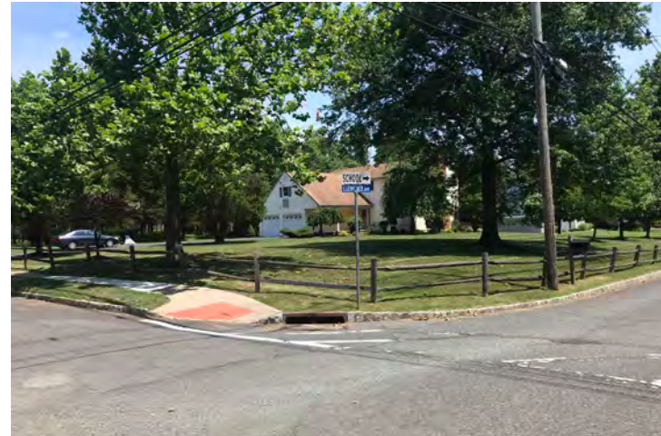
Curb cut and ramp are misaligned and too steep.
