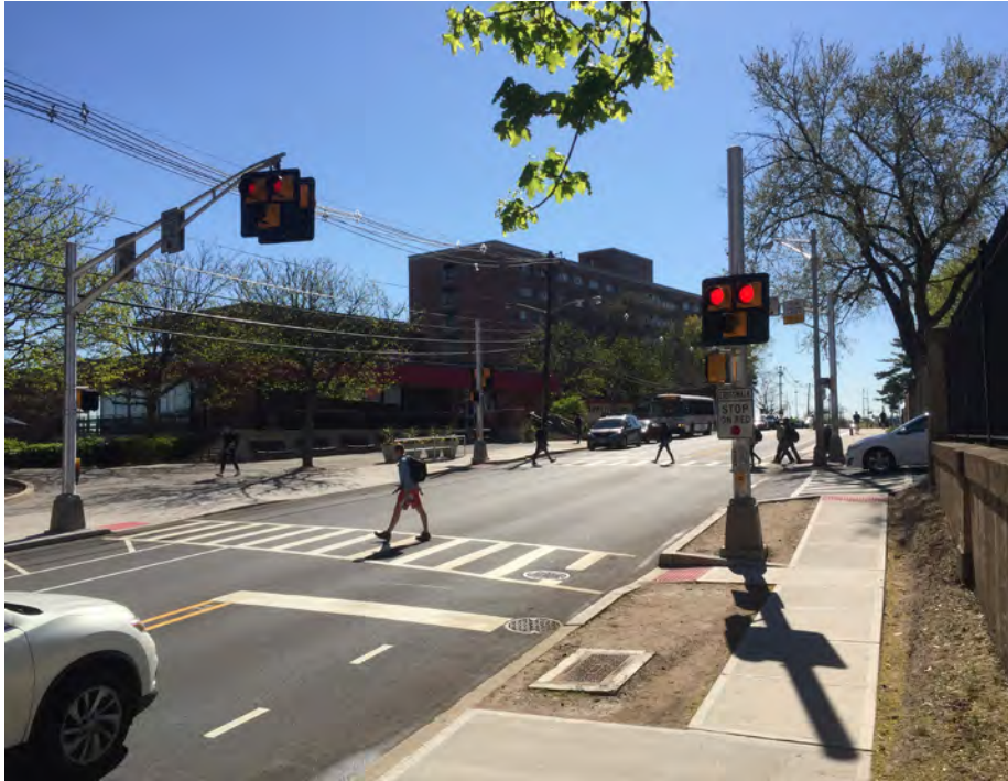
The HAWK signals on George Street in New Brunswick allow pedestrians to safely cross at mid-block locations.
