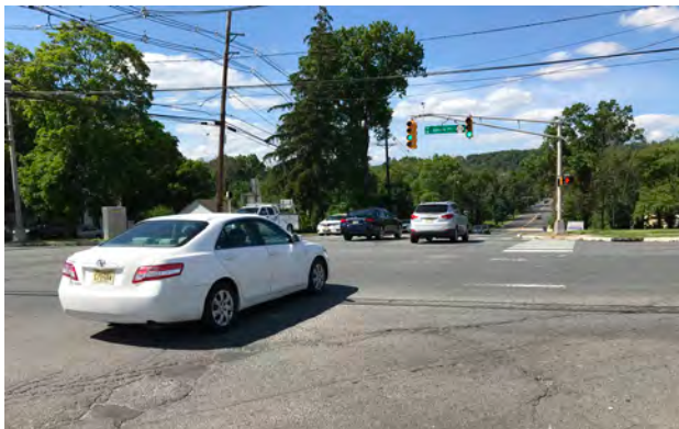
A crosswalk at the intersection of Union Ave and Finderne Ave is fading and difficult for drivers to see. This particular crossing is about 85 feet long.
