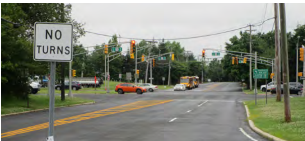
The busy intersection of Milltown Road and Route 22 includes just one crosswalk, located on the west side, that is not connected to any sidewalk.
