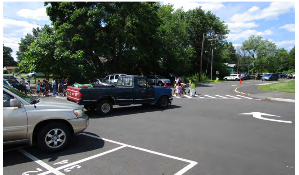
Cars entering and exiting the parking lot conflict with pedestrians using the Walter Street path, resulting in a potentially dangerous situation.
