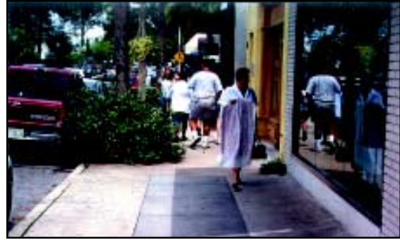
Figure 2.16: Less than five-foot clear width, Winter Park, Florida.
