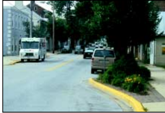
Figure A.2.5: East Main Street as reconstructed, Westminster, Maryland
