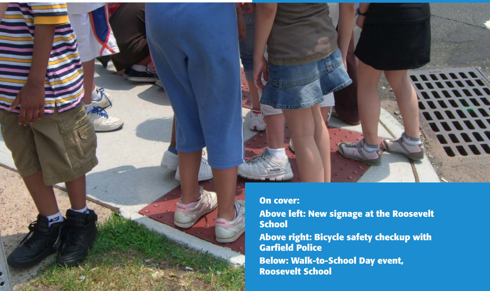
Below: New sidewalks with ramps and warning strips near Roosevelt School
