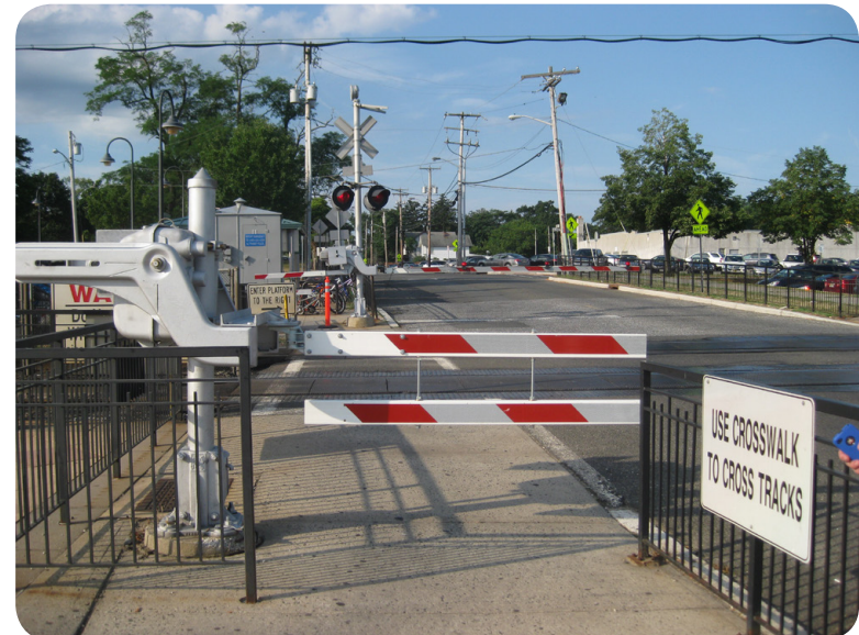
Pedestrian gate with “gate skirt” being tested at the Aberdeen-Matawan Train Station. Image: The RBA Group
