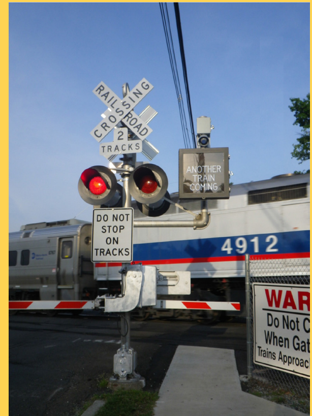
“Another Train Coming” system installed at Plauderville Station. Image: Marco DeSilva, Volpe Center
