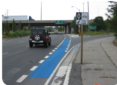
Providing bicycle facilities leading to and through the ramp improves visibility. Image: Cleanairpartnership.wordpress.org
