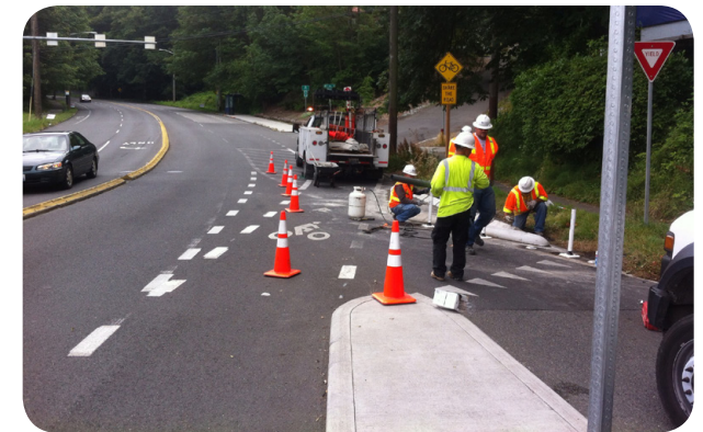
Seattle DOT installed a refuge median and curb extension at this right turn lane which narrows the travel way and forces motorists to slow down. Image: SeattleBikeBlog.com
