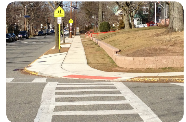
Diagonal curb ramps are not desirable because they force pedestrians into the intersection and are more difficult for visually-impaired people to determine the correct crossing location and travel direction. Image: Arterial
