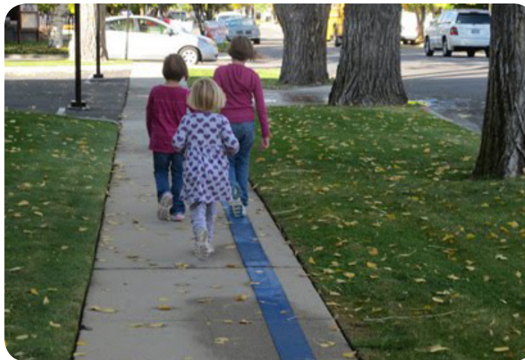
Carson City, NV marks its "Kit Carson Trail," with a six-inch wide, blue skid-resistant surface line. Image: RVfor5.blogspot
