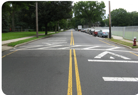
Raised crosswalk at Somerville School in Ridgewood, NJ. Image: The RBA Group
