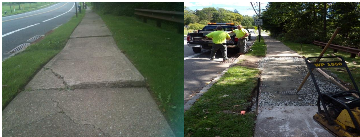
Photo: (Left) Deteriorating sidewalk/erosion on the southwest side of Southern Boulevard about 400 ft. east of SBS. (Right) Twp. Public Works Department making repairs during the summer of 2012.
