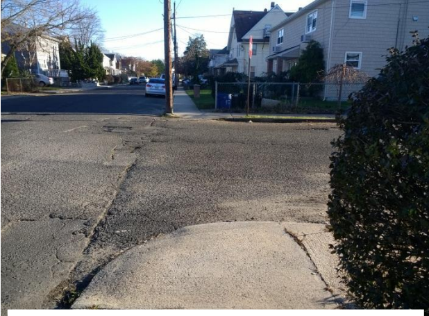
Missing/Faded Stop Bar
