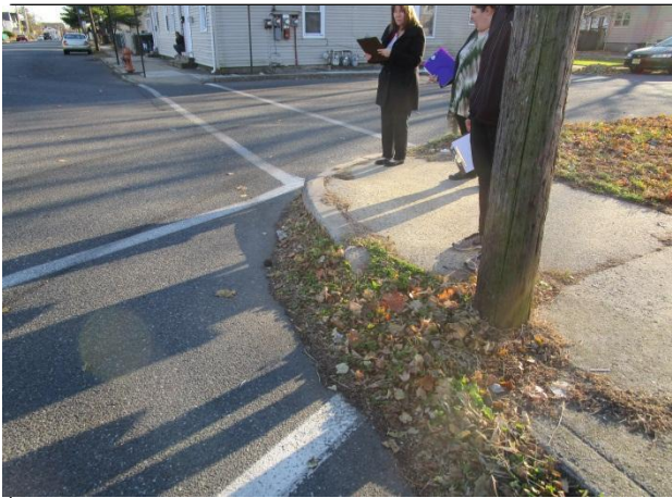
Broken/Missing Curb Ramp
