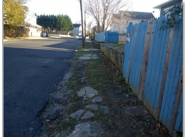
Broken/ Uneven Sidewalk
