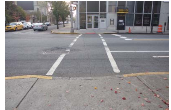
Missing truncated domes at West 26th Street & Broadway
