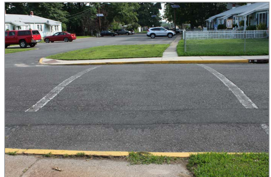
Missing curb ramps on Victory Dr near the entrance to Bellmawr Park Elementary
