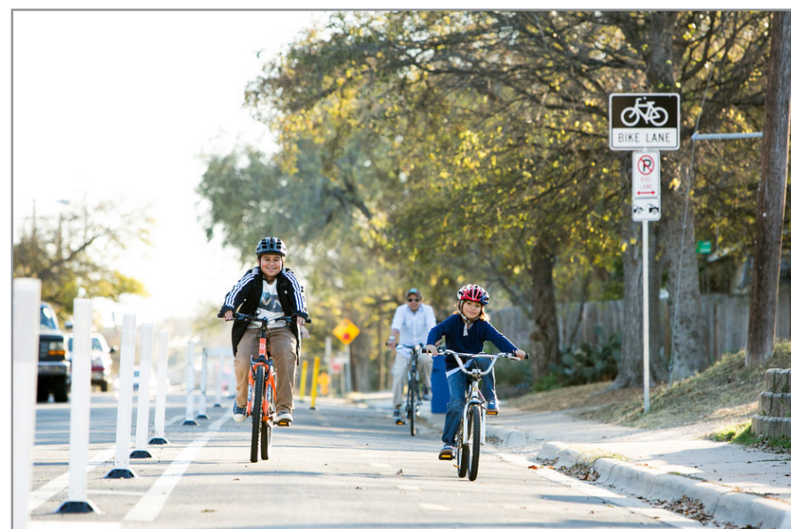
Flex posts added to the buffer to create a protected bike lane Credit: Green Lane Project
