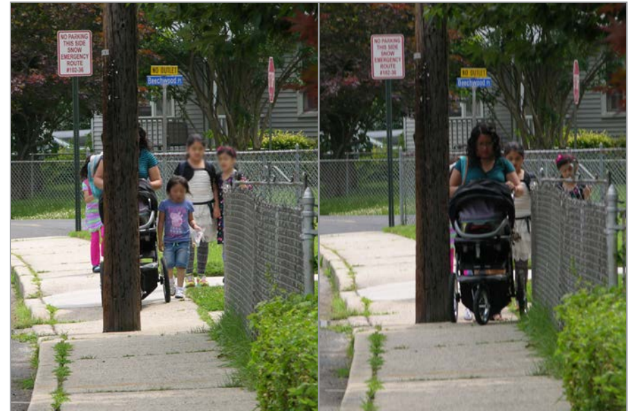
A pole on Victory Dr obstructs the path of travel for a mother walking with a stroller
