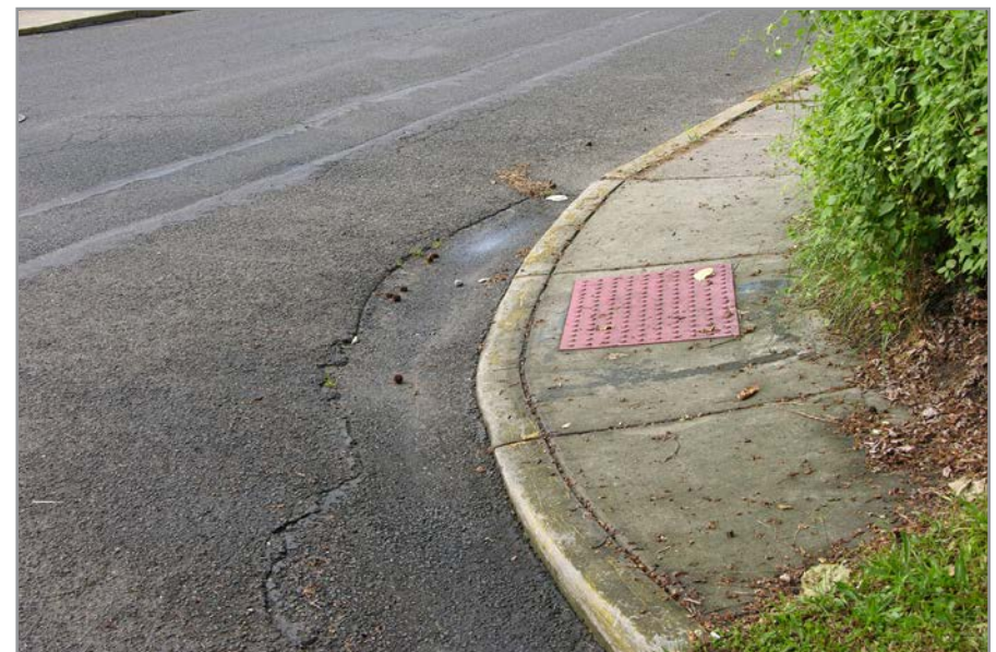
A poorly designed diagonal curb ramp
