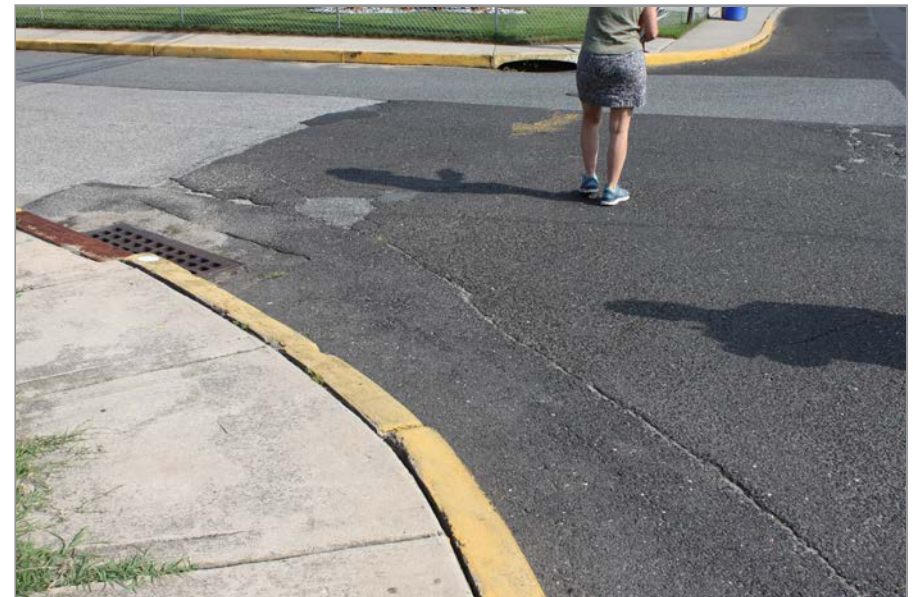
Missing curb ramps on Victory Dr
