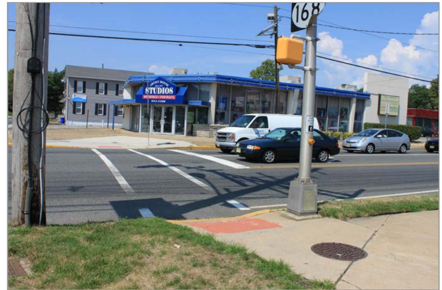
A standard crosswalk begins to wear down on the Black Horse Pike
