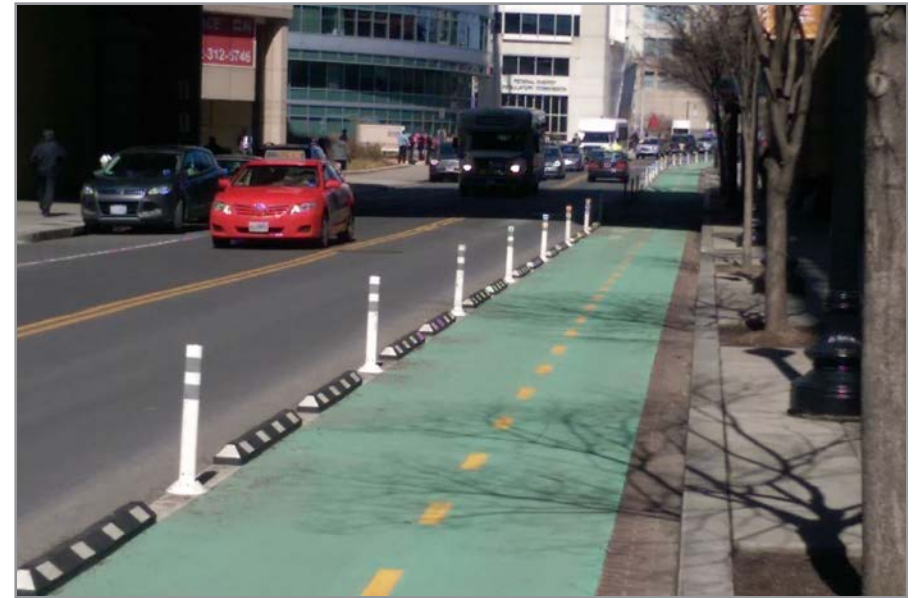
A two way protected bike lane in Washington DC using curb stops and flex posts
