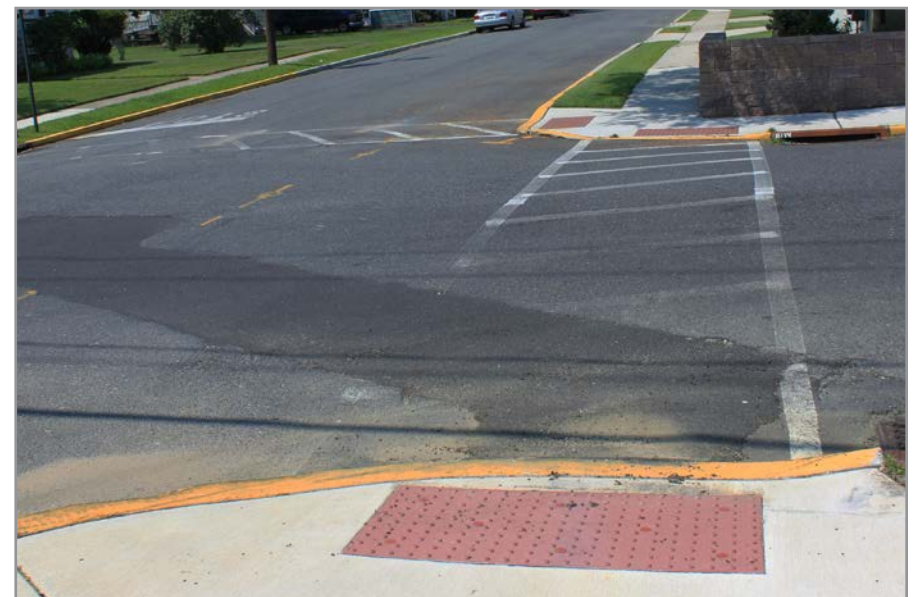
ADA compliant curb ramps on Lowell Ave, near E.M. Burke Elementary
