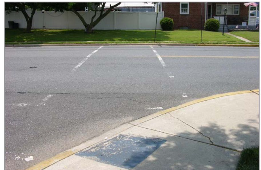
A badly faded standard crosswalk spanning Creek Road at Bell Rd
