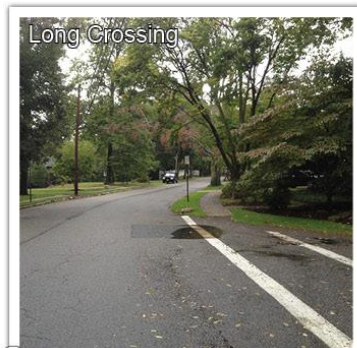
4 The pedestrian crossing is minimally defined, very long and lack curb ramps.
