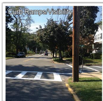
16 This crossing has no curb ramps and drivers cannot see pedestrians due to the utility pole.
