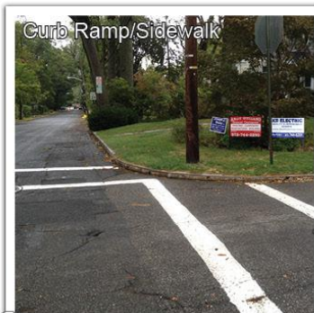
5 Crosswalks are provided but there are no curb ramps or landing areas on the connecting corner.
