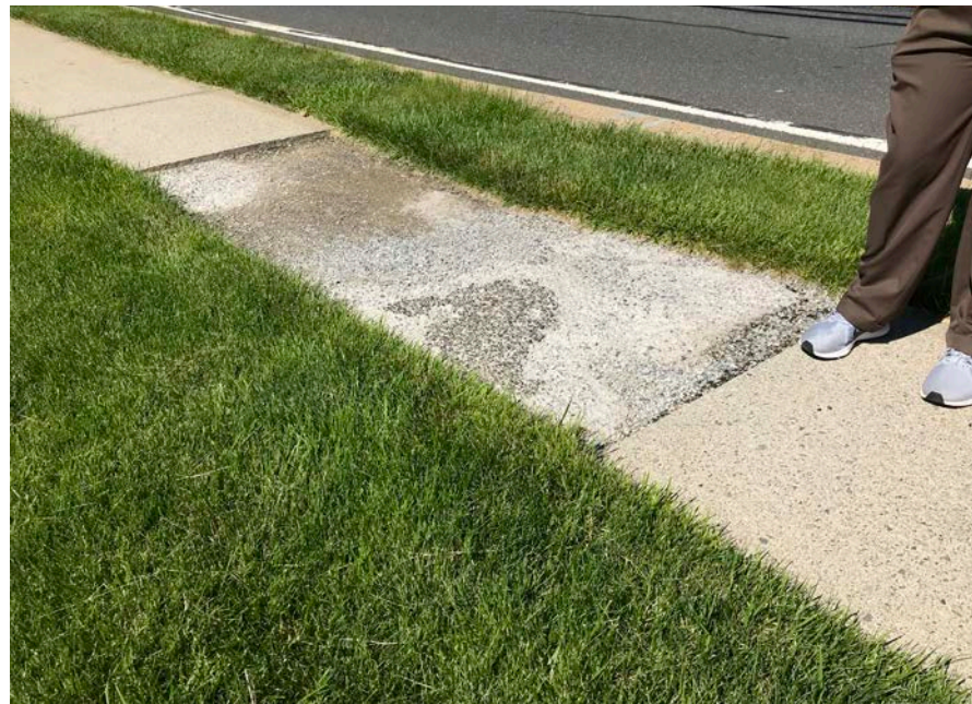
Deteriorating sidewalks and plant growth has resulted in inaccessible crossings along North Bridge Street (near 3rd Avenue)
