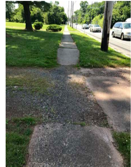
Sidewalk deterioration along Finderne Ave (left) and Union Ave (right) reduces accessibility.
