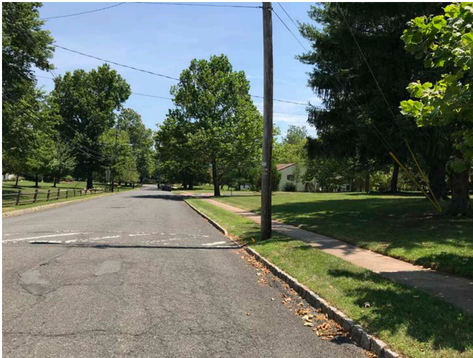
A faded crosswalk on Steeplechase Lane leads directly into a utility pole and does not connect with the sidewalk.
