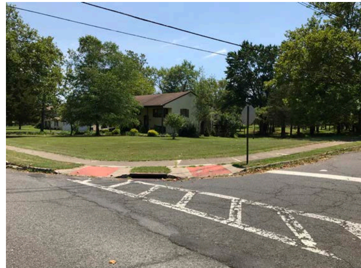
Duplicated curb cuts and warning pads make crossing confusing and dangerous. (Intersection of Farmer and Steeplechase)
