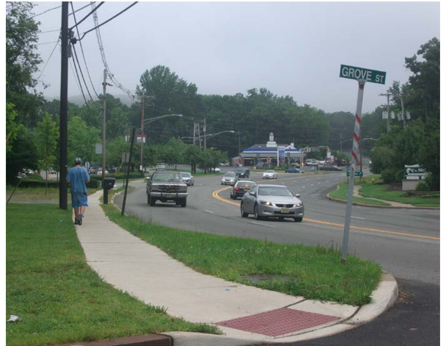
Unobstructed sidewalks with buffers and curb ramps improve pedestrian accessibility and mobility, especially along busy roadways. (Source: SRTS Resource Center)
