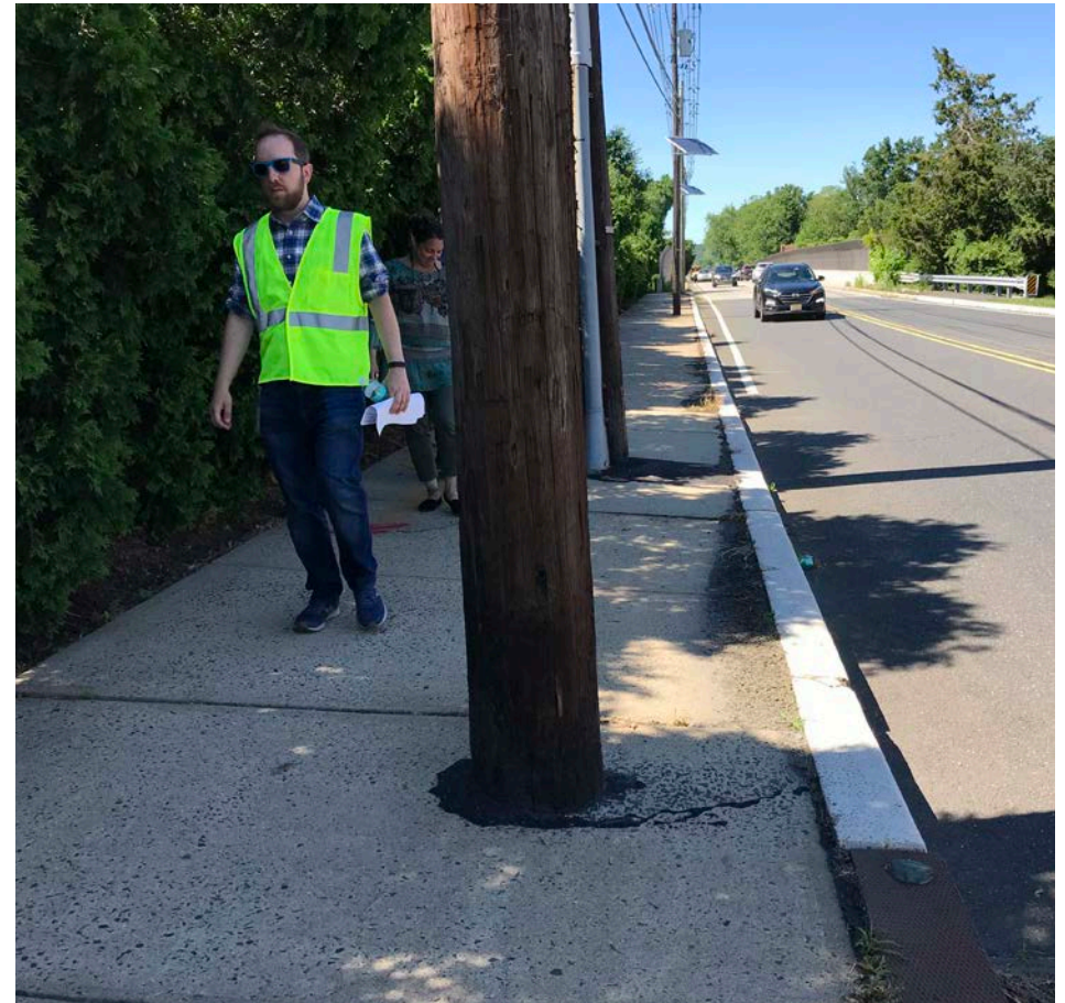
Sidewalk on North Bridge Street interrupted by utility poles, reducing safety and accessibility
