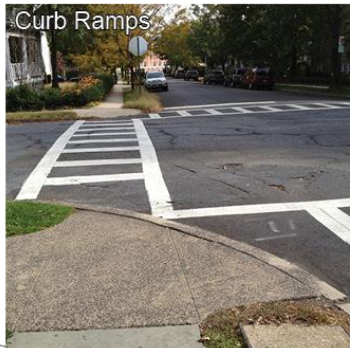
10 Proper curb ramps are not provided at this intersection.
