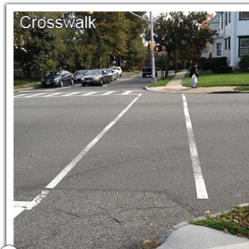
2 Crosswalks are faded and not highly visible.
