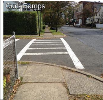
12 Proper curb ramps are not provided at this intersection.
