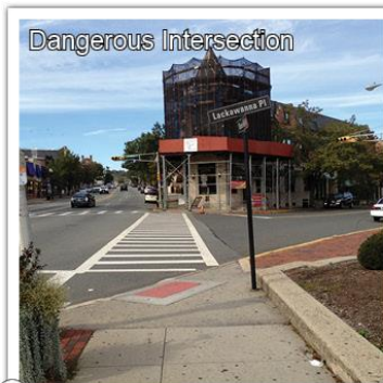
7 Long crossing distance and current roadway alignment allowing cars to make this turn at high speeds make for a dangerous pedestrian crossing.
