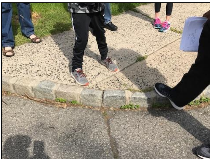
Non-sloped sidewalk on Cook Ave. missing a curb cut and truncated dome.
