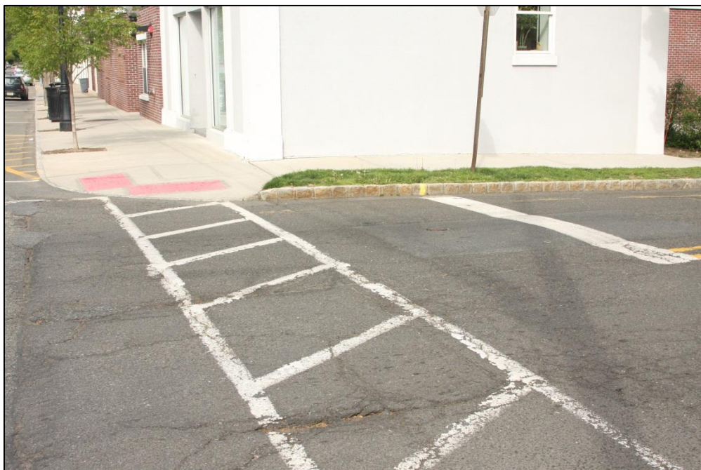
Crosswalk at Central Ave. and Elmer St. is faded and street cracked
