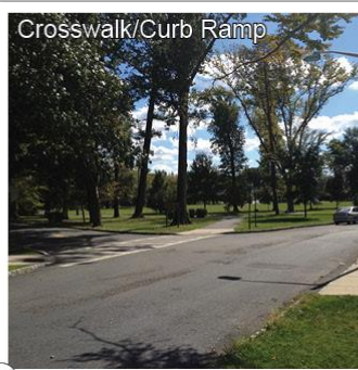
2 No safe crosswalk or curb ramp is provided from west side of Edgemont Road.
