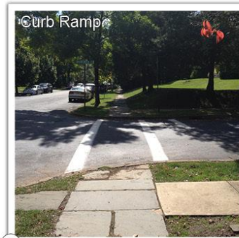
12 Intersection lacks curb ramps and corners are in poor condition.
