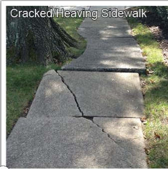
3 There are some areas of cracked and heaving sidewalks along Edgemont Road.
