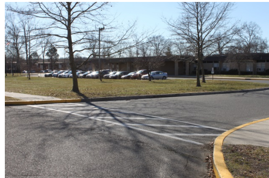
Figure 8: Entrance at Busansky not equipped with ADA-compliant curb ramp
