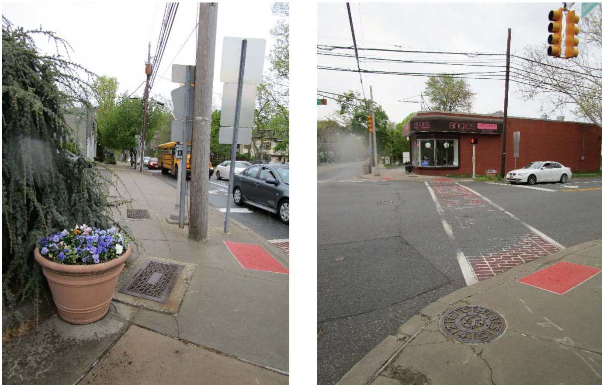
Figure 21 - Amboy Ave. at Main St. – sidewalk obstructions and worn crosswalks
