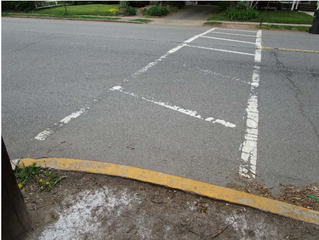
Figure 7 - Lack of curb ramps and pole obstruction at Main St. at Talmadge Ave.
