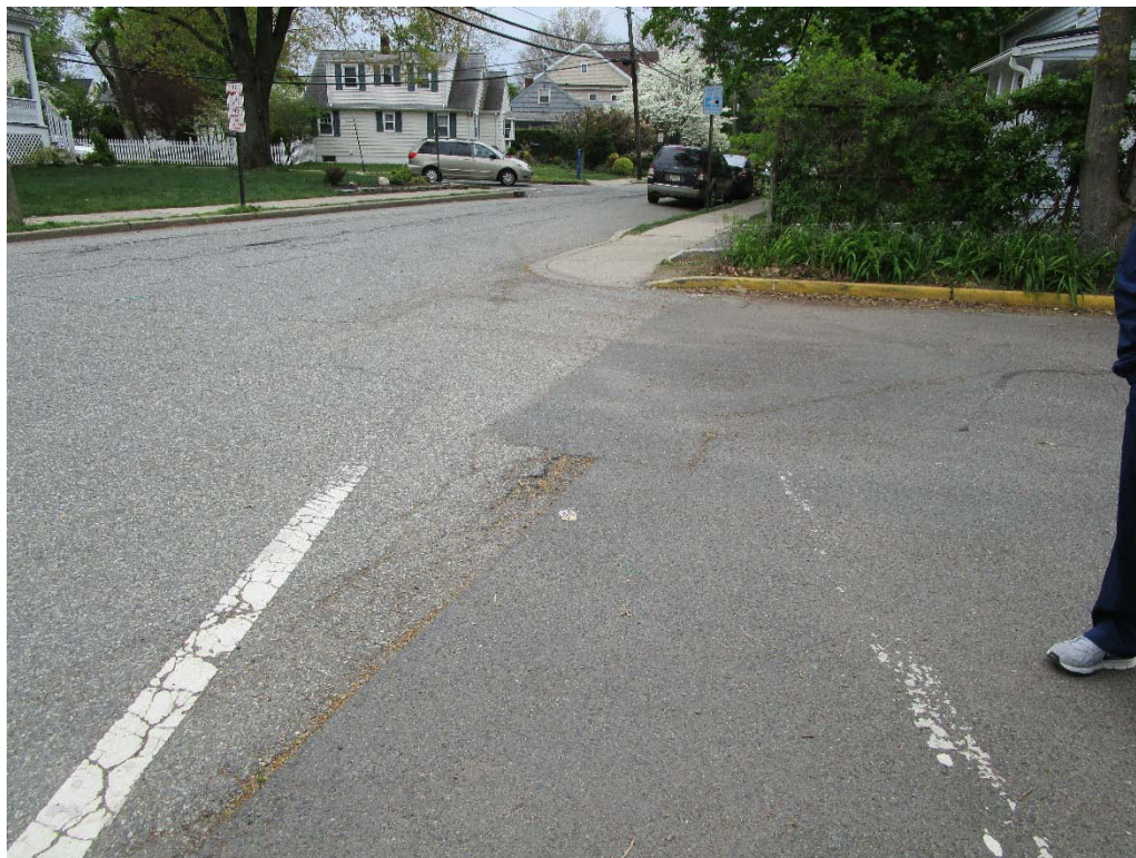
Figure 7 - Crosswalk paint wear
