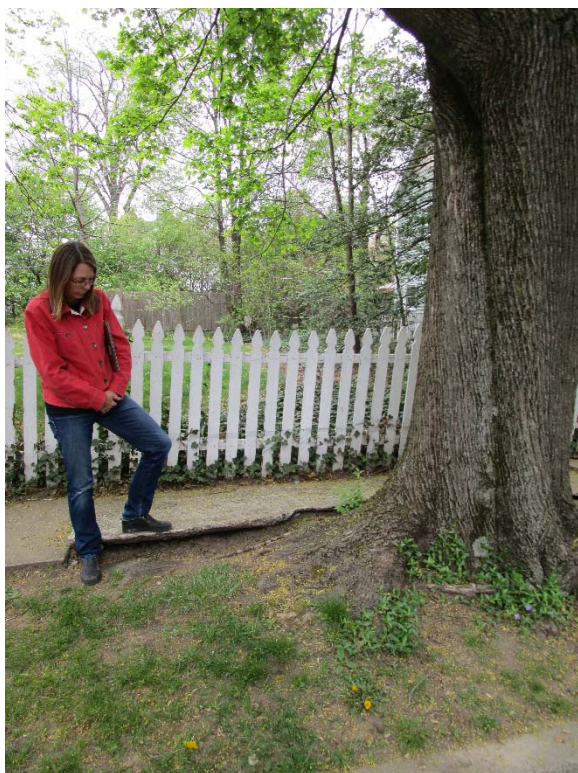
Figure 19 - Sidewalk uplift on Thomas St. (left); sidewalk slope on Spring St. between Lake and Graham (right)
