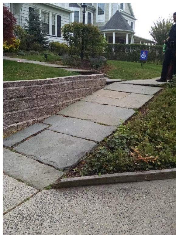
Figure 19 - Sidewalk uplift on Thomas St. (left); sidewalk slope on Spring St. between Lake and Graham (right)
