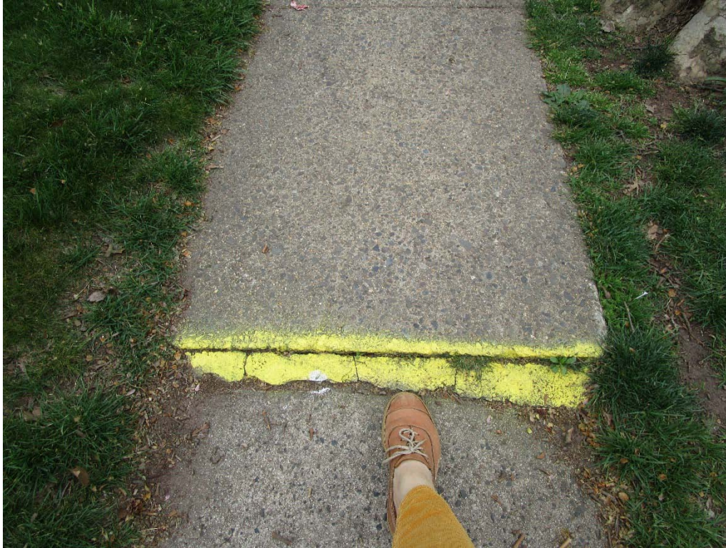
Figure 11 - Uplifted sidewalk
