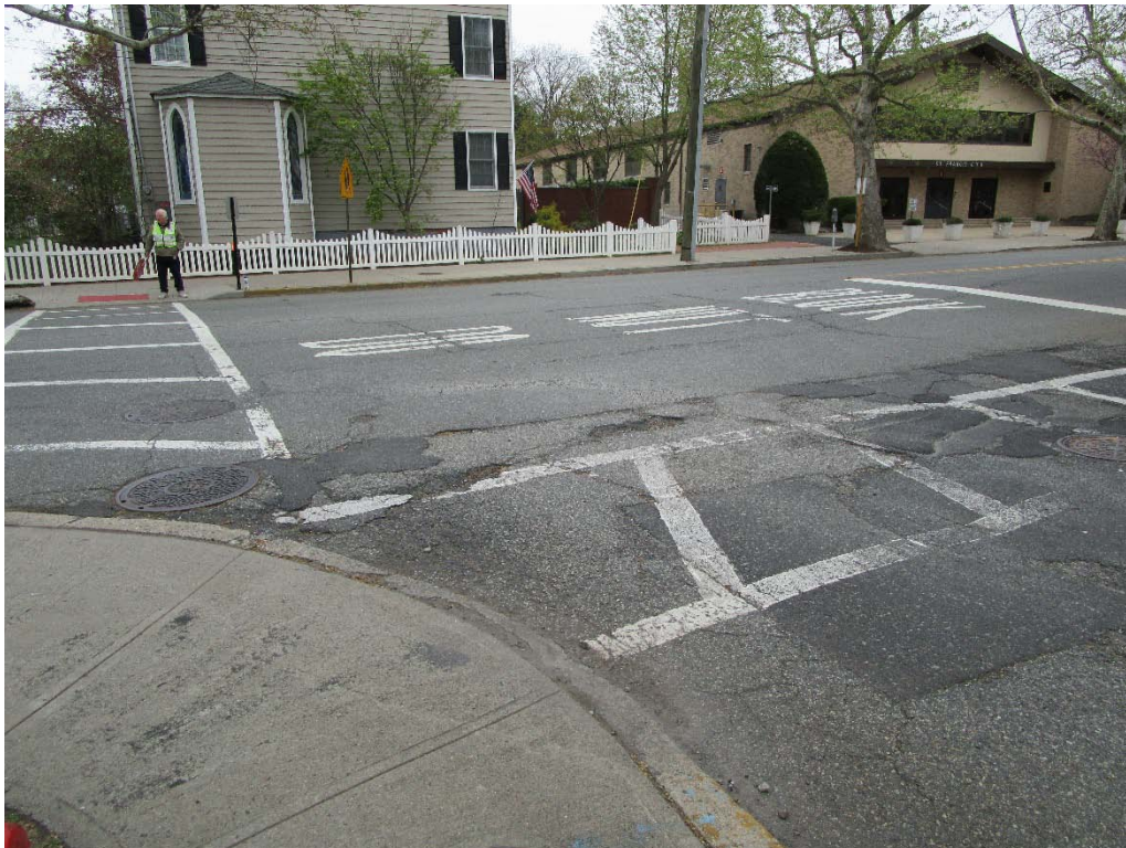
Figure 10 - Pavement condition in crosswalks at main St. at Durham Ave.
