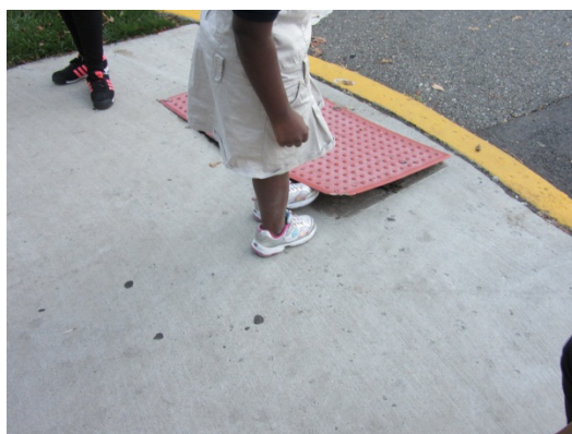
Image 13 Broken Truncated Dome on 3rd Street
