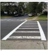
Curb ramps and corner conditions at this connection point to the school and the park are crumbling and not ADA compliant.
