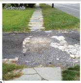
9 Sidewalk is cracked and crumbling at driveway apron.
