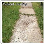
Sidewalks in this area are cracking and crumbling in some locations.
