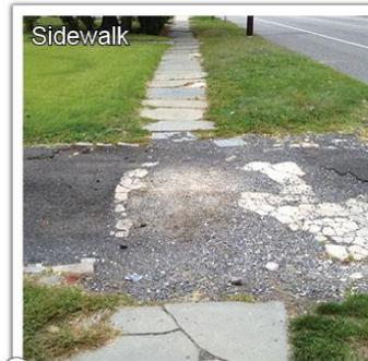
9 Sidewalk is cracked and crumbling at driveway apron.
