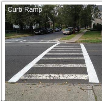
5 Curbs ramps and corner conditions at this connection point to the school and the park are crumbling and not ADA compliant.
