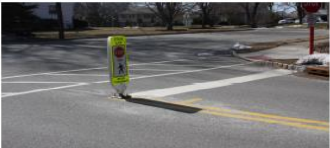
Newly painted crosswalk and stop line. Permanent "Stop for Pedestrians in Crosswalk" sign
