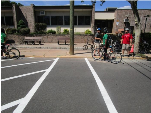
Figure 18 – A utility pole obstructs a crosswalk on Mansfield St. at Grove St.
