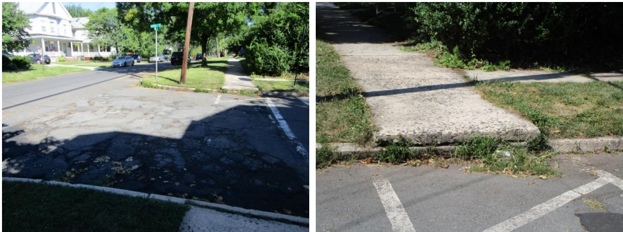
Figure 11 - Poor pavement condition and high curb at S. 3rd Ave. at Harper Pl.
