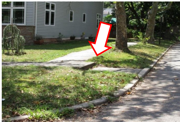
Figure 4 - Step on sidewalk on Donaldson St. & S. 3rd Ave.
