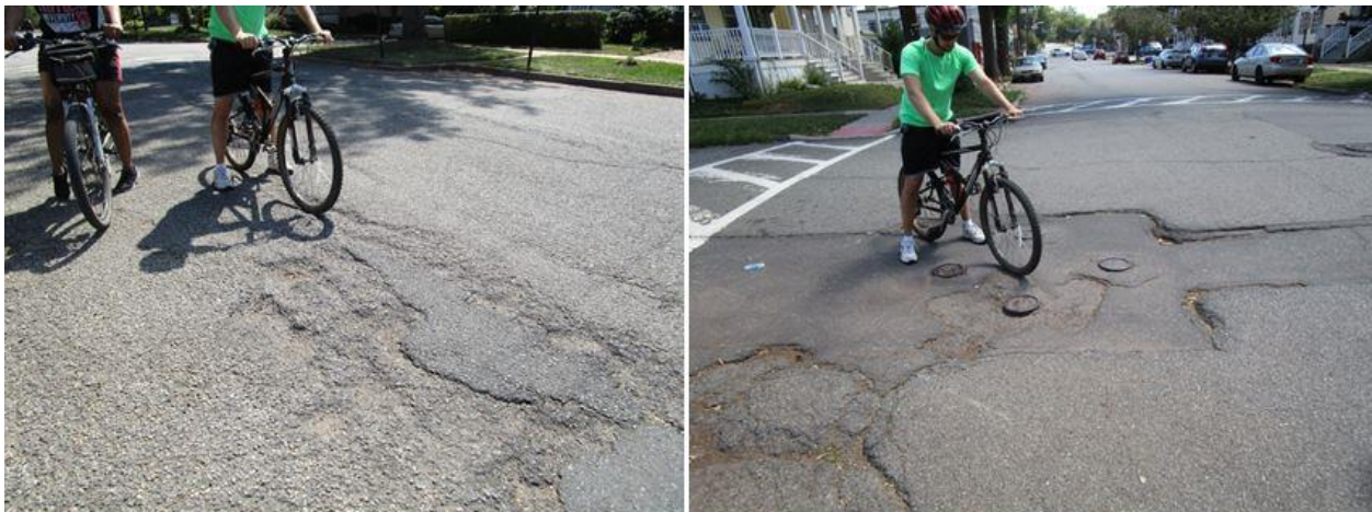
Figure 19 - Poor pavement condition from potholes and patching.
