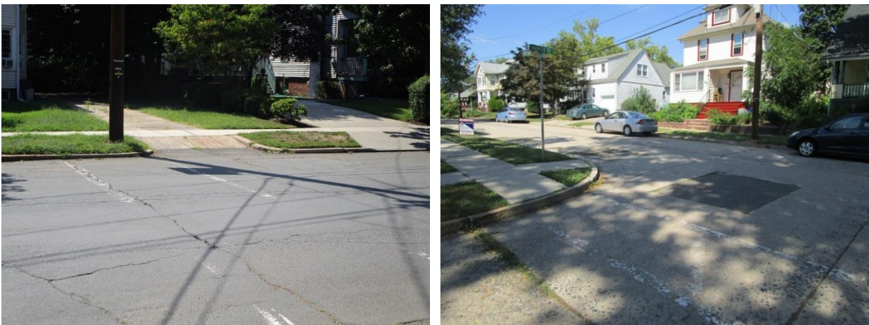
Figure 12 - Faded crosswalks and lack of curb ramps at S. 1st Ave. at Magnolia St. (left) and Felton St. at Harper Ave. (right)
