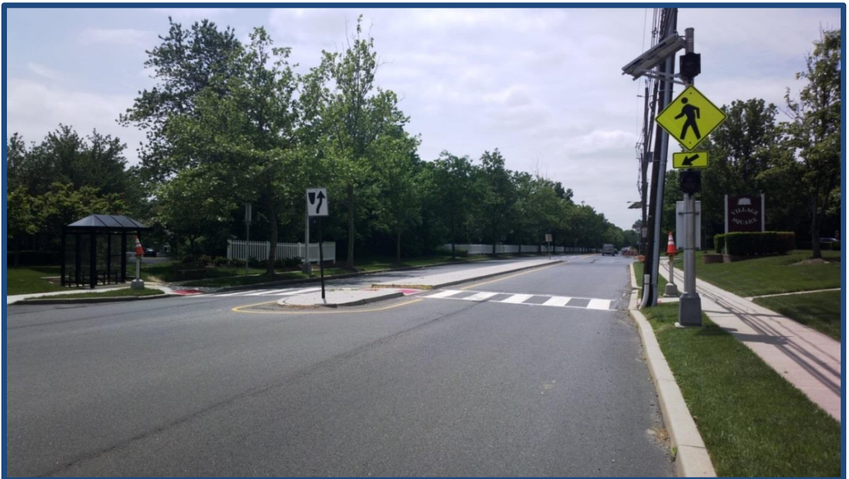
Above from Clarksville Rd, CR638, West Windsor - the flashing beacon has incandescent lights and a regular, up and down blinking pattern in one direction.
