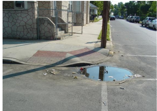
Drainage issues impede crosswalk at the intersection of Hayes Avenue and Beideman Avenue
