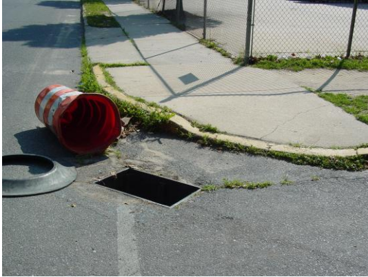
Open utility chamber impedes the crosswalk at the intersection of Hayes Avenue and N. 31 st Street near Camden's Promise
