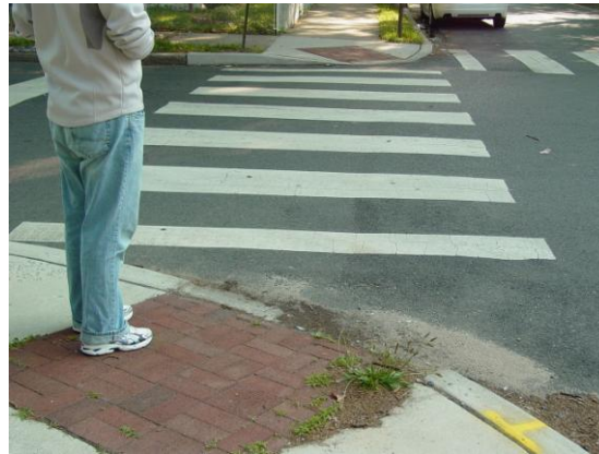
High visual crosswalk striping pattern, apex ramp with brick pavers – no tactile warning
