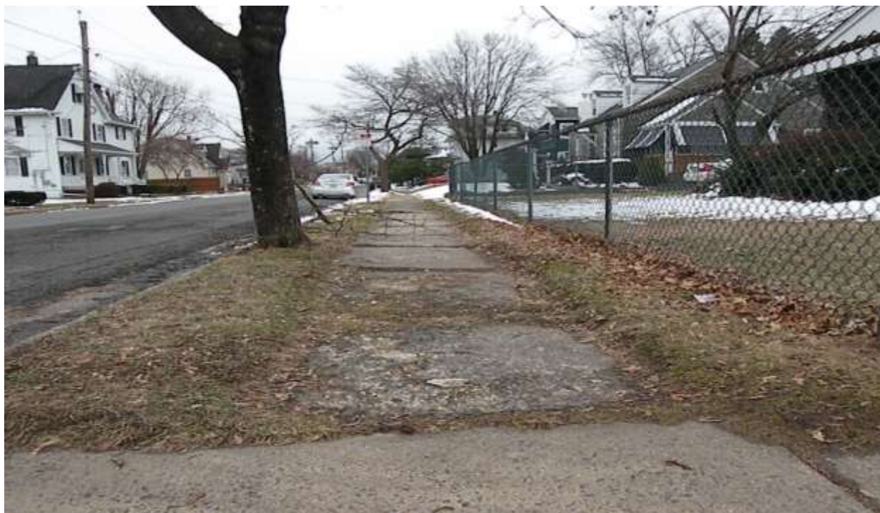
Cracked and partially blocked sidewalk.
