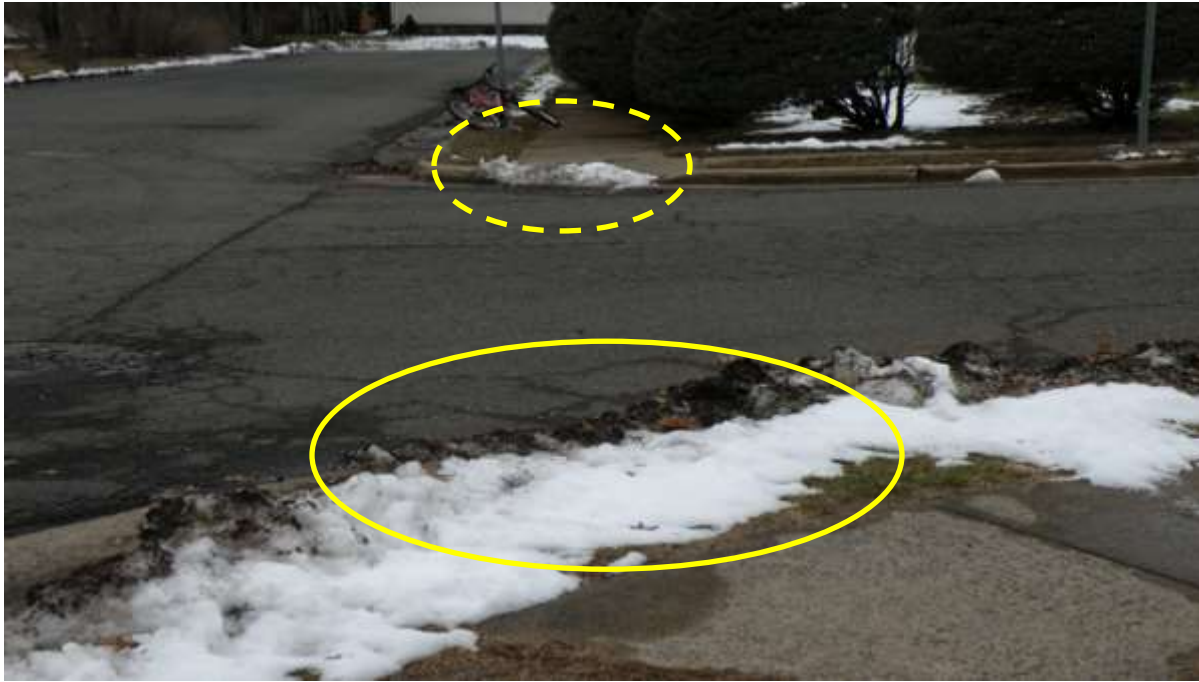
Missing curb cut on opposite corner with snow removal issue in the curb cut.
