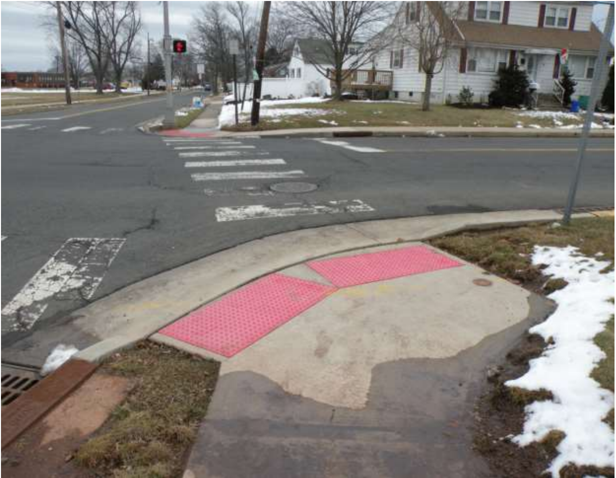
New curb ramps with ped head at N.13 th & Brooks Blvd
