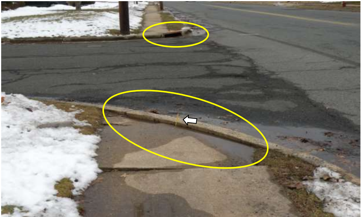
Curb drop with pencil highlighting perspective with catch basin on opposite corner preventing installation of a curb cut.
