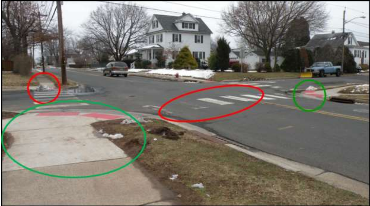
Work in progress - new sidewalks and truncated domes with faded crosswalks and snow removal issues, Brooks Blvd & N.9 th Ave.
