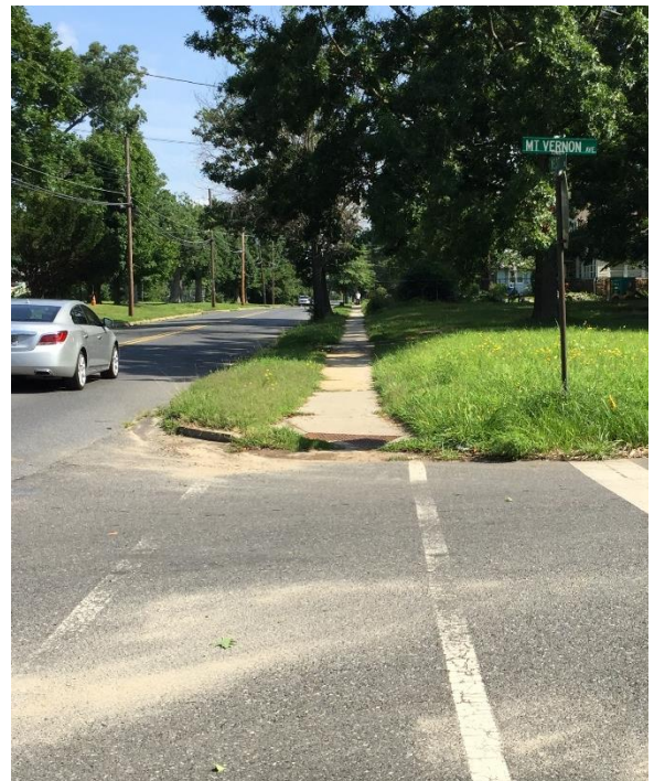
Figure 9. West Avenue & Mt. Vernon Avenue - Non-compliant handicap ramp
