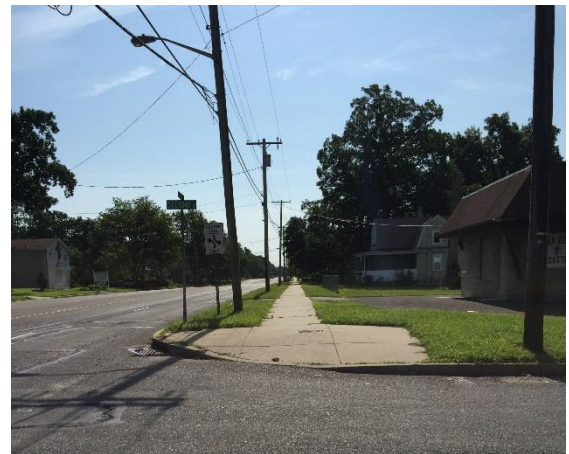
Figure 14. Park Avenue & 2nd Street - Non- compliant handicap ramp
