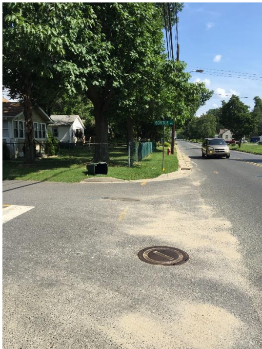
Figure 8. West Avenue & Bortle Avenue - Missing sidewalk and ramp
