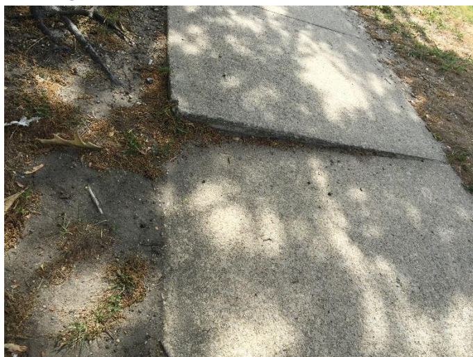
Figure 15. Chestnut Ave. - Uneven Sidewalk
