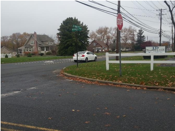
Figure 31. Main Rd. & Washington Ave. – No Crosswalk, missing sidewalk, no ramp
