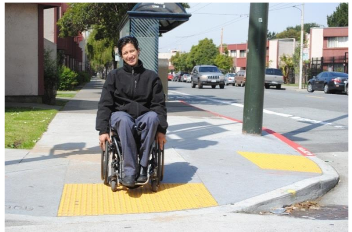
Figure 35. Handicap Accessible Sidewalk Ramp
