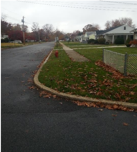
Figure 32. Embassy Terrace & Linda Ave. – No Crosswalk, missing sidewalk, no ramp
