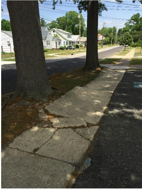
Figure 23. Columbia Ave. (East side) - Uneven sidewalk
