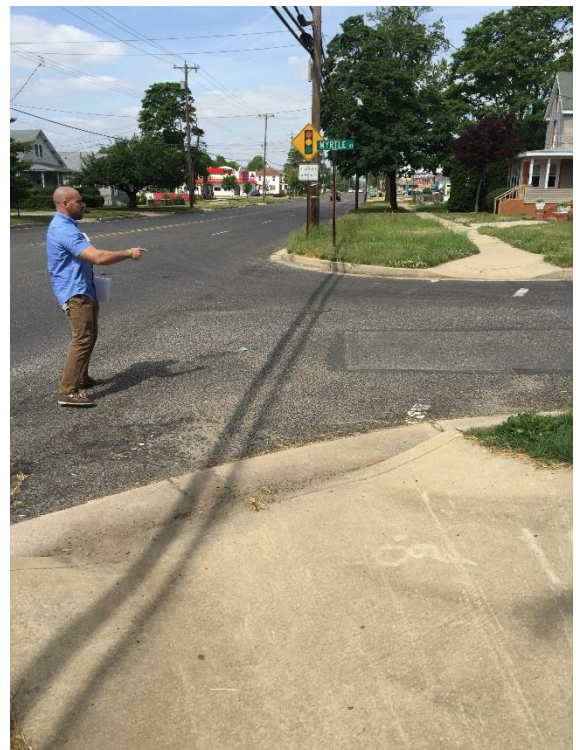
Figure 13. Chestnut Ave. & State St. Non- ADA compliant sidewalk ramps and faded crosswalk
