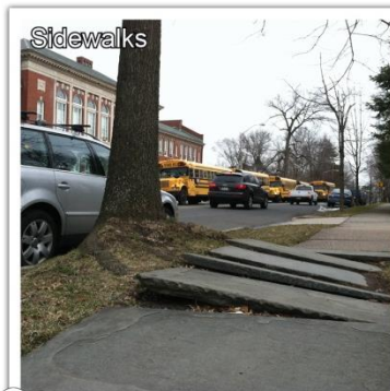
5 Some sidewalks around the school are old slate walks and are cracked and heaving.
