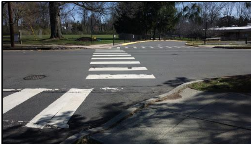
Riverside Dr and Robert Rd- Level the steep curb grade, add ADA pad
