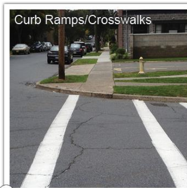
7 Intersection improvements are needed including curb ramps and corner landings.
