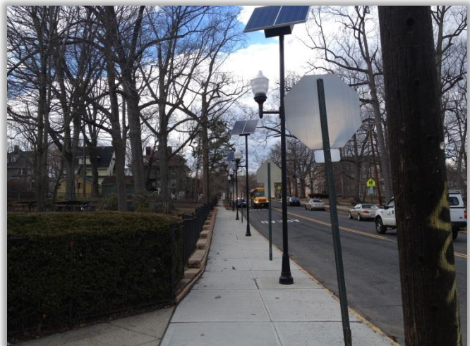
New solar-powered pedestrian scale lighting, sidewalk and retaining wall
