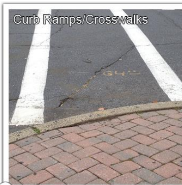
8 Curb ramps needed (along most of this street).
