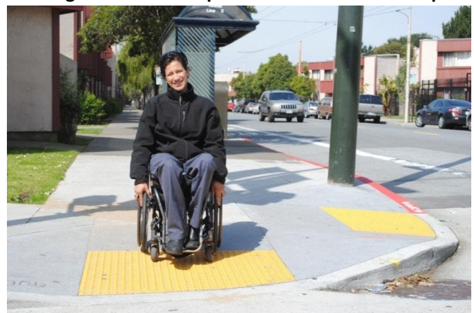
Figure 18. Handicap Accessible Sidewalk Ramp
