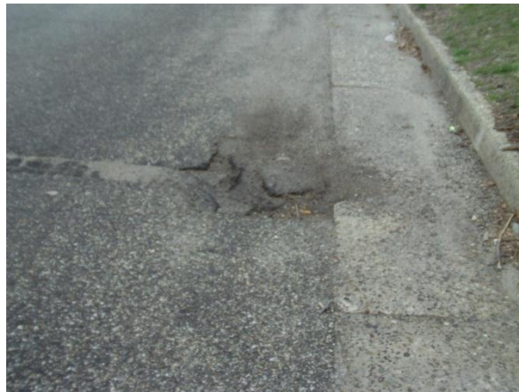
Figure 14. Grape Street -Untreated Pothole
