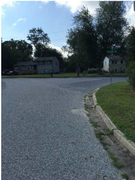
Figure 17. Venus Drive - Missing crosswalk, missing sidewalk, and missing shoulder.
