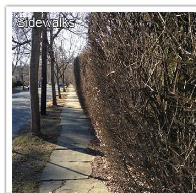
7 Sidewalk along this side of Garden Street is old, cracked slate and has overgrown shrubs obstructing sidewalk width.
