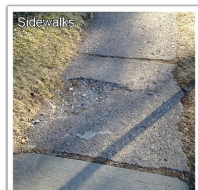
9 Sidewalk is sufficient but is cracked and heaving in many locations.
