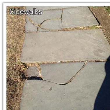
5 Many of the sidewalks on side streets are the original slate and are cracked and heaving.
