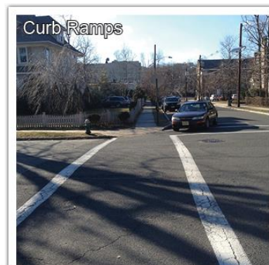
4 Good intersection but lacks truncated dome paver ramps. Also, the standard "ladder" crosswalk used around the school would be more visible.
