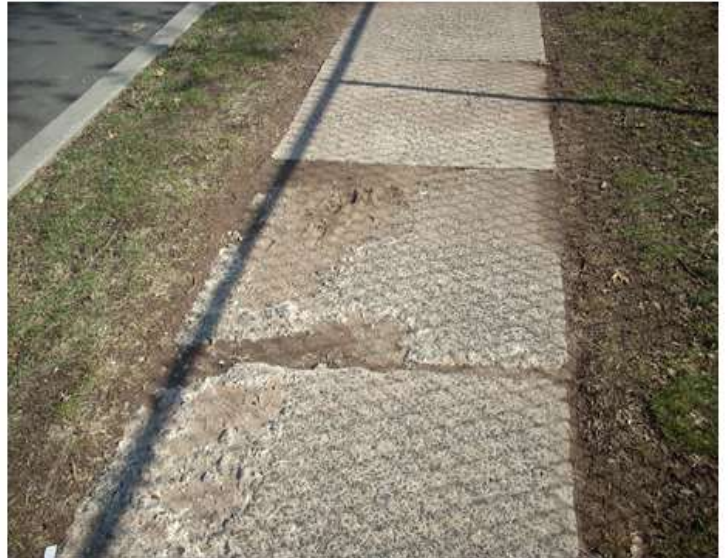
580' of Sidewalk in front of West End School needs replacement. 120'replaced in Summer of 2011.
