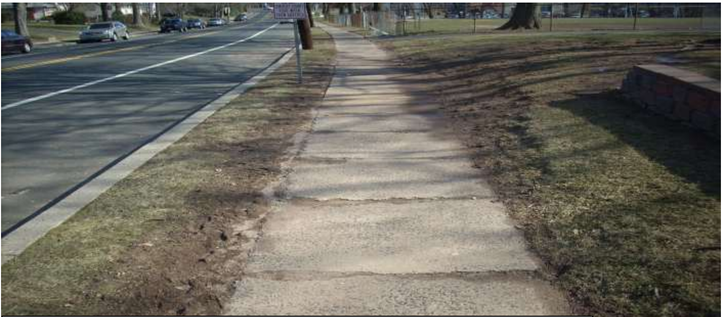
580' of Sidewalk in front of West End School needs replacement. 120'replaced in Summer of 2011.
