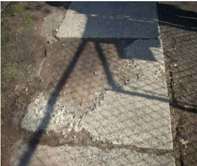
580' of Sidewalk in front of West End School needs replacement. 120'replaced in Summer of 2011.
