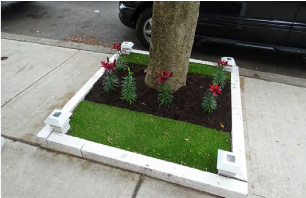
Street Tree with Tree Filter box in Jersey City
