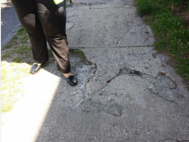
Cracked, Uneven Sidewalk
