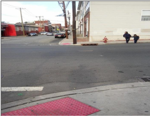
Misaligned Truncated Dome Pad
