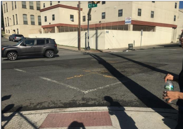
Misaligned Truncated Dome Pad directs blind pedestrians into the intersection, not the crosswalk
