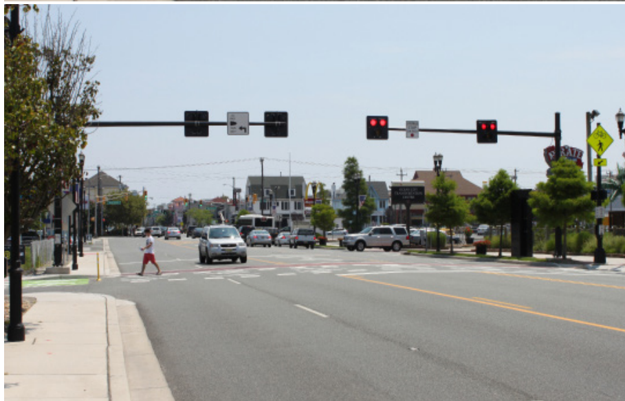
A HAWK in operation in Ocean City, New Jersey
