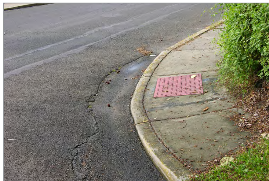
A poorly designed diagonal curb ramp
