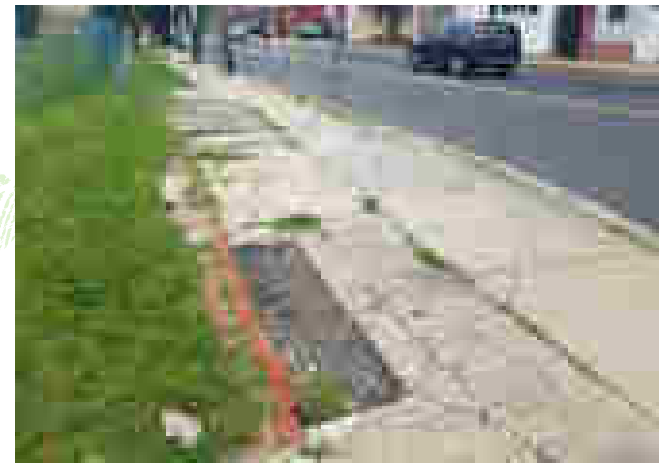
Heavily damaged sidewalk with utility box frames protruding from concrete on Talmage near West Main Street. Picture provided by Ridewise, Inc.
