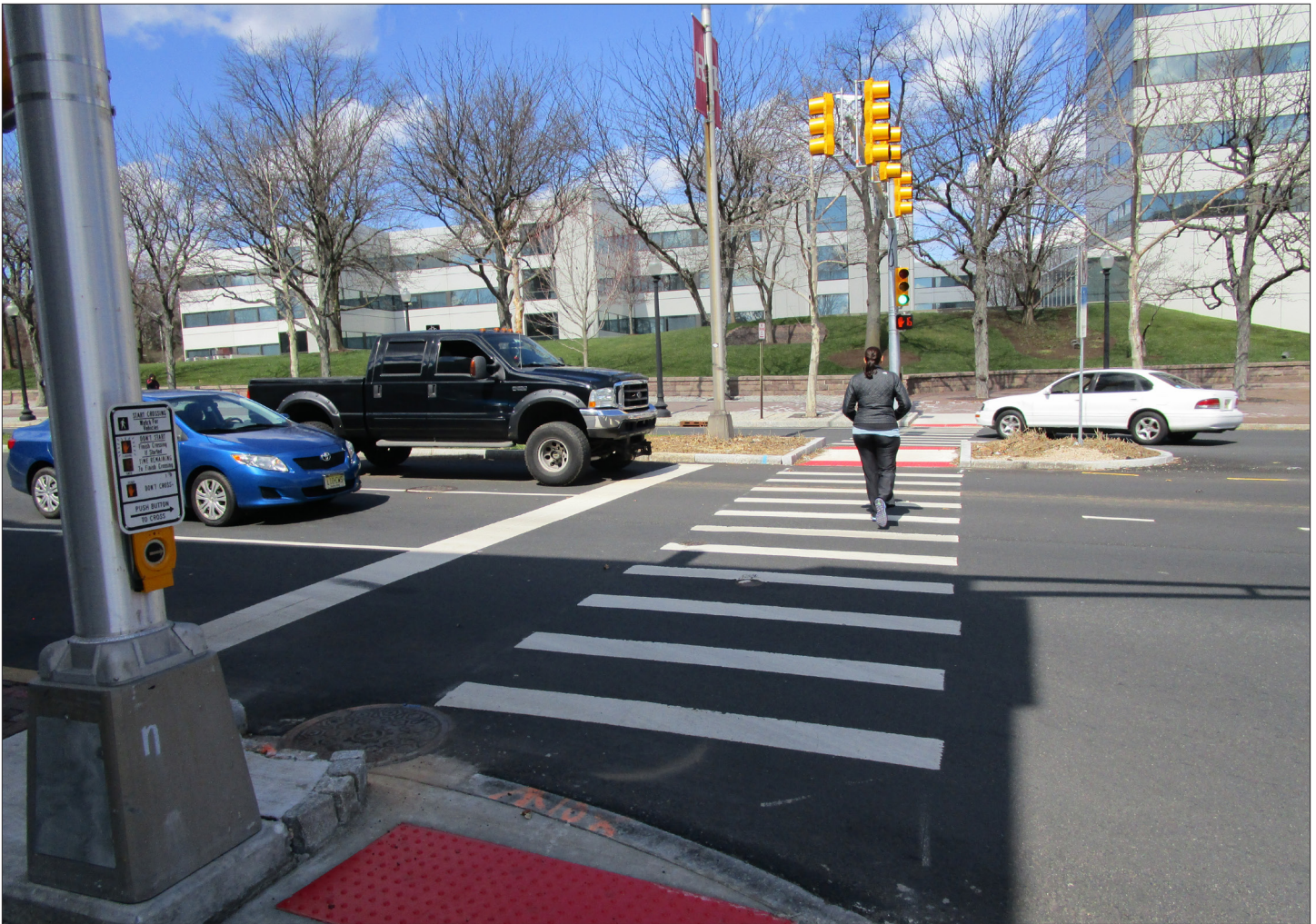
High visibility markings improve crosswalk visibility compared to transverse lines.
