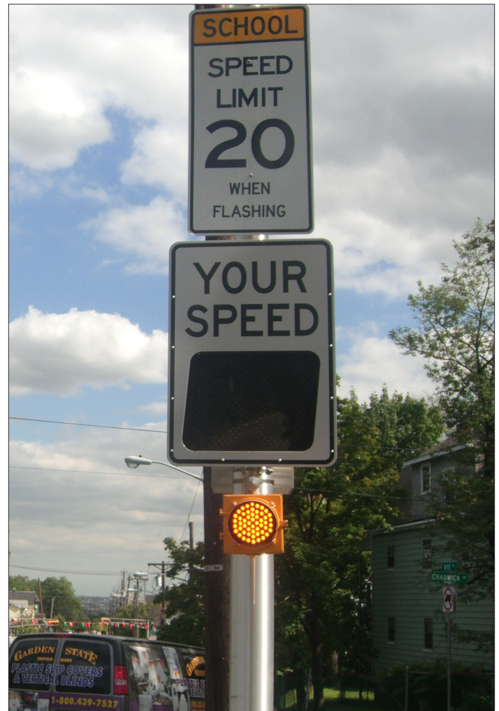
Speed monitoring displays in school zones, especially those with text and flashing lights, are effective in both the short- and long-term.
