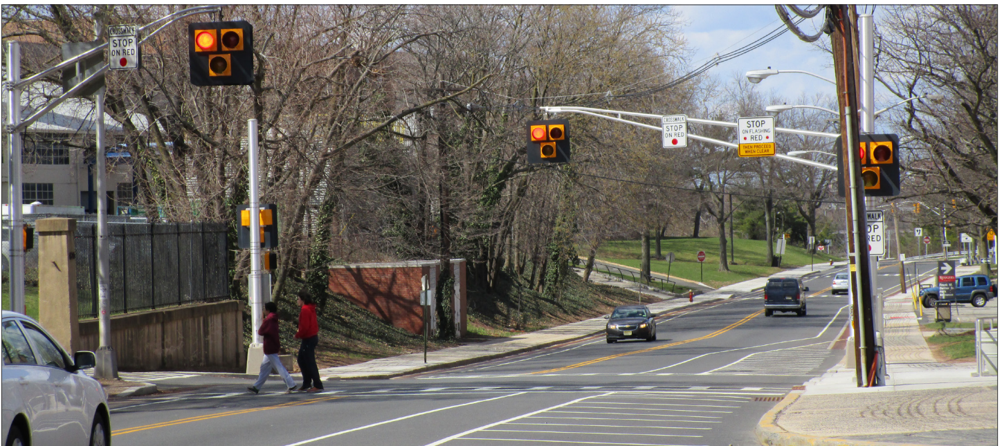
Pedestrian Hybrid Beacons can reduce pedestrian crashes by assigning right of way and providing positive stop control.
