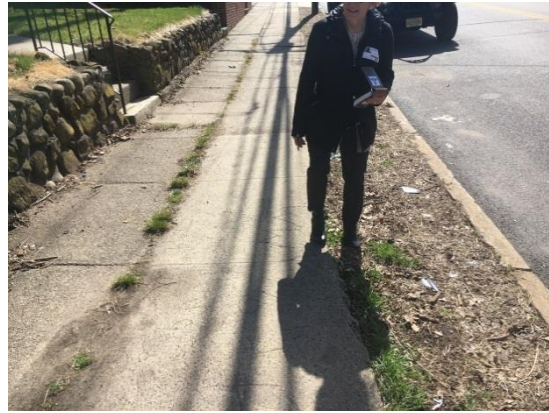
Weeds growing in cracks are unsightly and may damage sidewalk eventually
