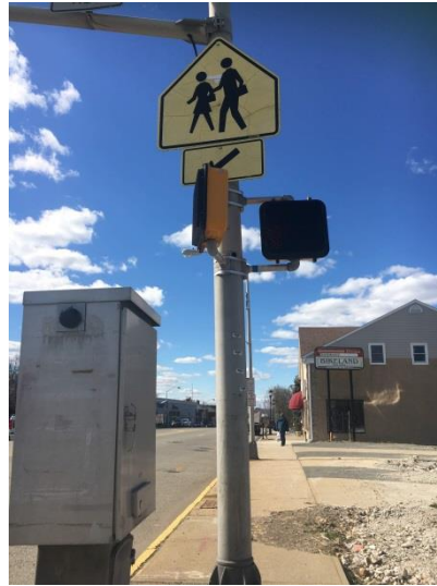
Central Ave. & Bloomfield Ave. Signal post and signal box both obstruct sidewalk
