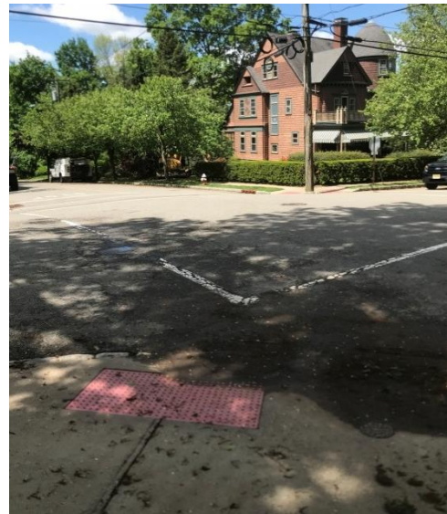
Crane St. & Arlington Ave. Misaligned dome pad directs blind into intersection instead of crosswalks. Add lighting at corner as shaded
