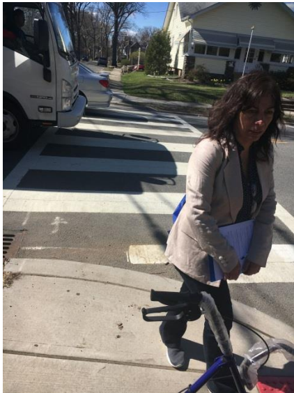
Central Ave. & Wakefield Place New crosswalk missing ADA dome pads
