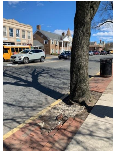
Bloomfield Ave Tree roots are starting to uproot the brick tree wells and sidewalk
