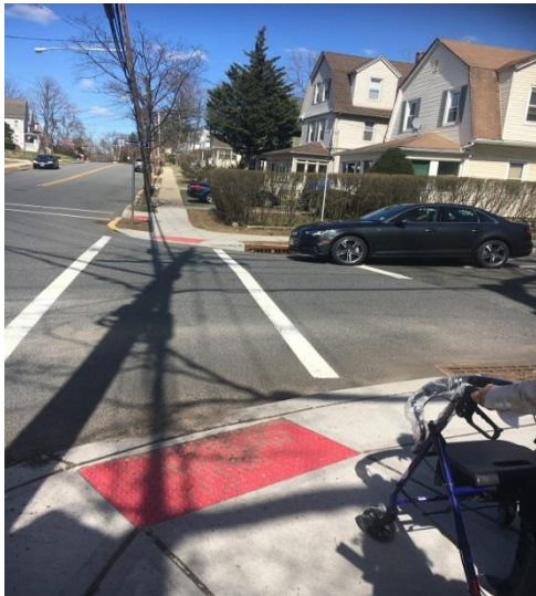
Central Ave.& Whitfield Ave. Misaligned dome pads and lack of high visibility crosswalks
