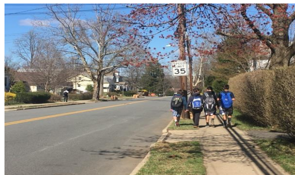
Wide lanes on Central Ave. do not have shoulders and encourage speeding beyond the posted limit of 35 mph. Investigate if bike lane or shoulder can be added to slow traffic
