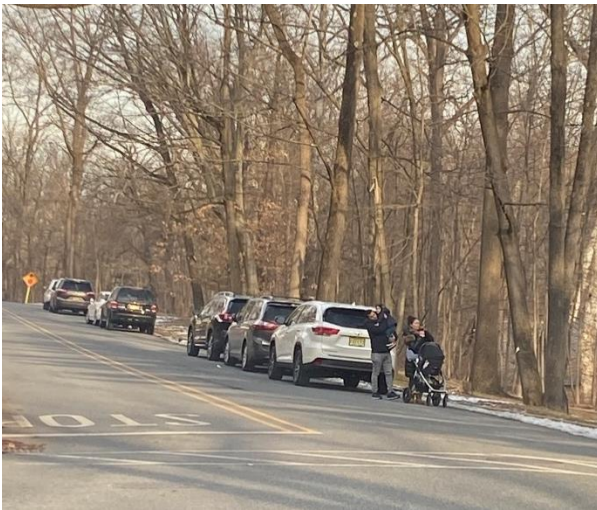
Gould Place & Brookside Ave. Crosswalk is faded and is very hard for drivers to see. Suggest to repaint with thicker lines
