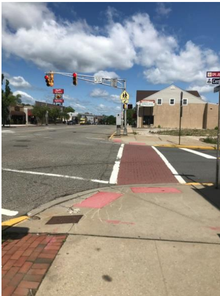
Bloomfield Ave. & Central Ave. (looking across Central Ave) Faded crosswalk. Suggest to repaint as high visibility crosswalks. Good signage and ped signals
