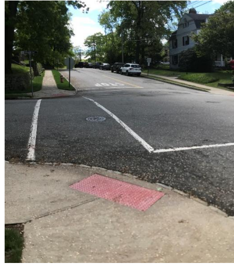
Arlington Ave. & Crane St. Misaligned dome pad. Add high visibility crosswalks
