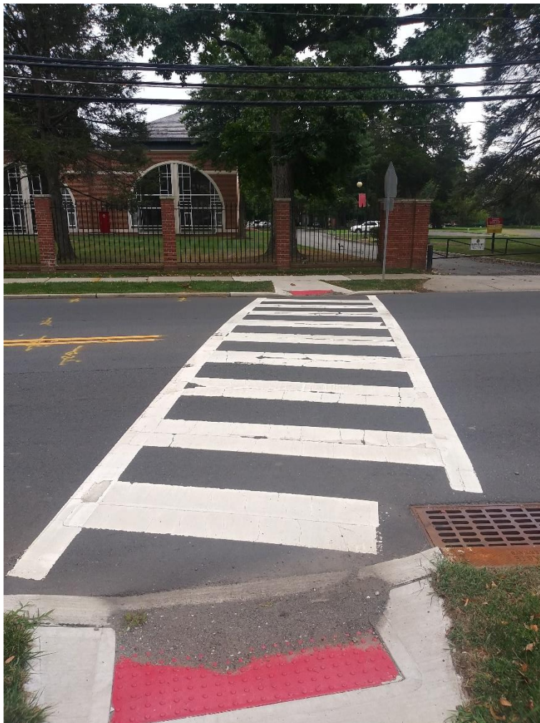
Figure 1 Uneven crosswalk level leads to debris being collected on ADA bump pad.
