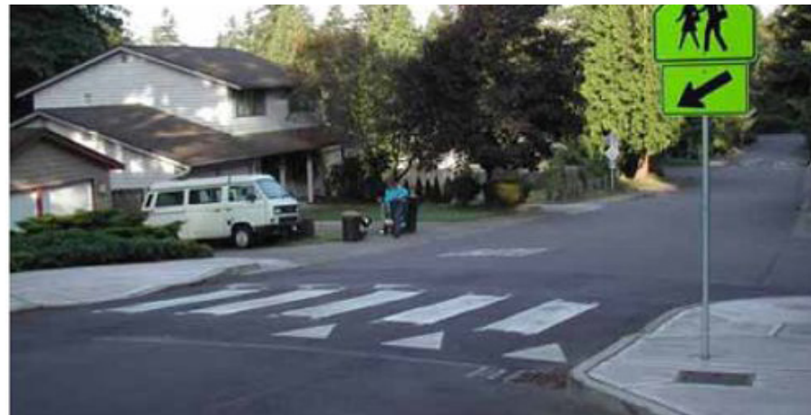
Figure 6: Curb Extensions and Speed Table Paired to Form a Raised Crosswalk
