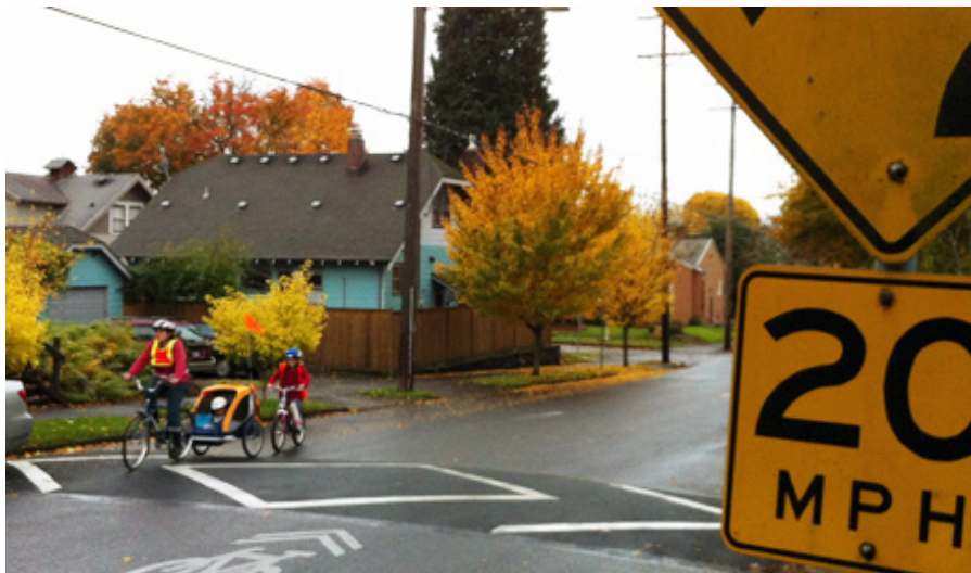
Figure 7: Example of a Speed Hump Used on Bicycle Boulevard
