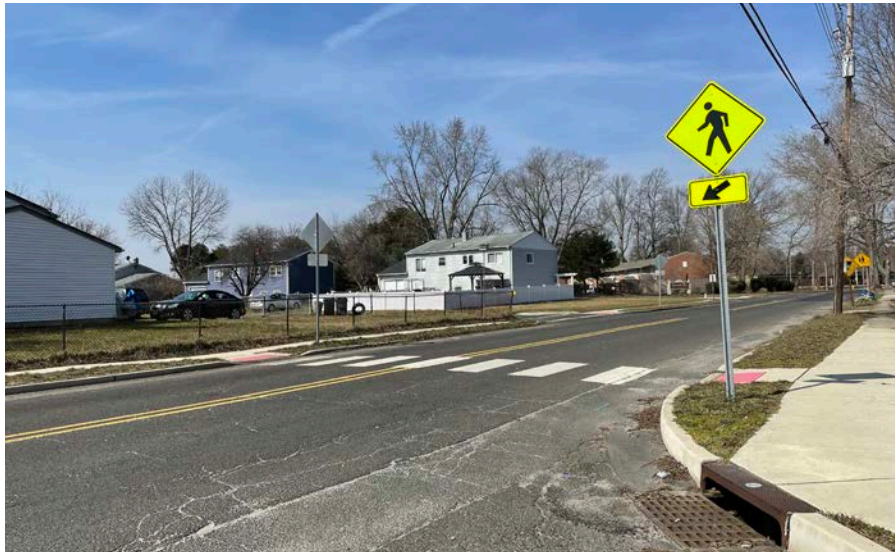
Figure 3: ADA-Compliant Curb Ramps at Harvard Avenue
