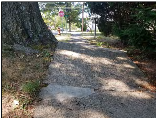
Picture 4: Sidewalk Damaged by Street Tree on Columbia Ave
