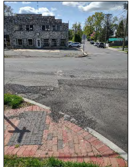
Picture 26: Missing Crosswalk and Sidewalk at Broad St and Greenwood Ave Intersection (Photo Taken from Northeast Corner)
