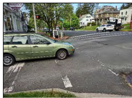
Picture 25: Faded Crosswalk at Broad St and Greenwood Ave Intersection (Photo Taken from Southeast Corner)
