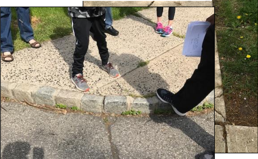
Non-sloped sidewalk on Cook Ave. missing a curb cut and truncated dome. t St.
