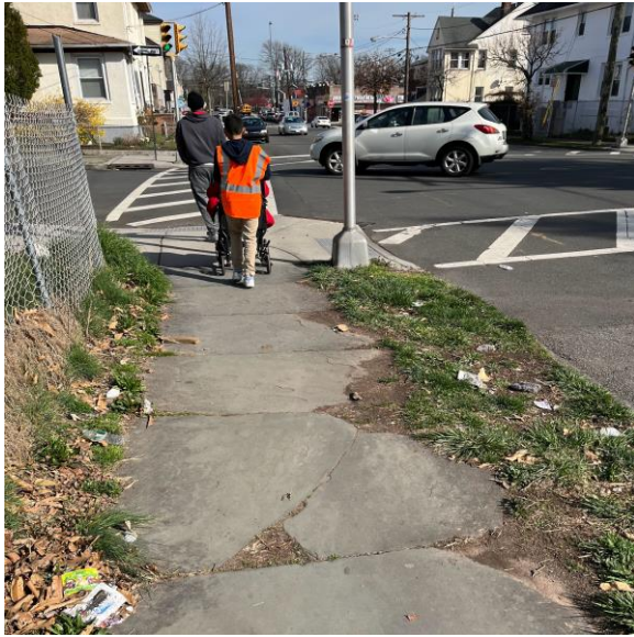
Sidewalk is uneven, cracked, and absent Intersection of 3rd Ave. & N. 7th St.
