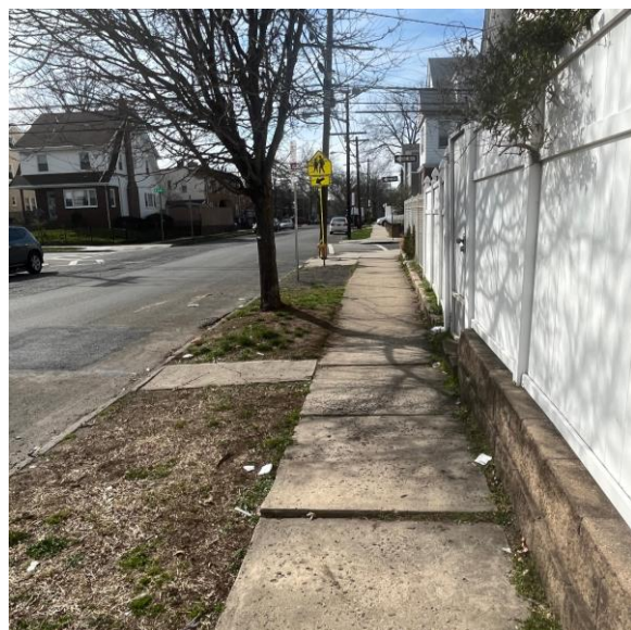
Sidewalk not level, tripping hazard and hard for wheelchairs/strollers 2nd Ave.
