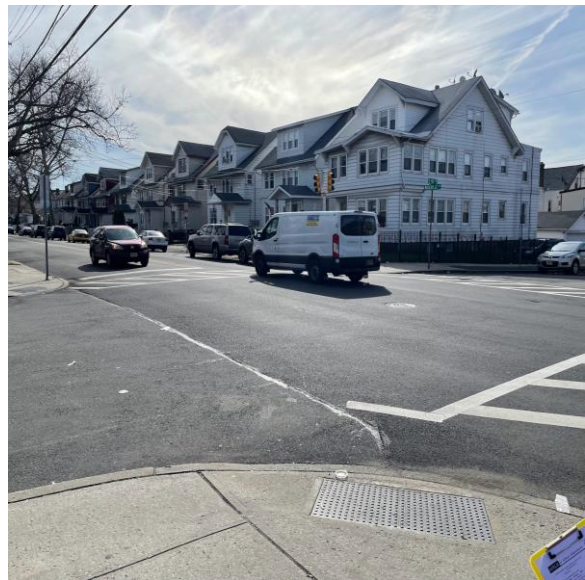
No crosswalk on the left and dome pad facing toward the middle of the intersection Intersection of 2nd Ave. & Roseville
