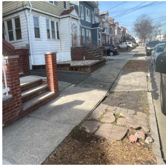
Sidewalk uneven when meeting driveway, driveway very cracked & uneven N. 11th St.
