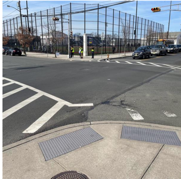
Crosswalk present in one direction but other is faded, dome pads are misaligned and direct the blind into traffic at 1st Ave. & Roseville
