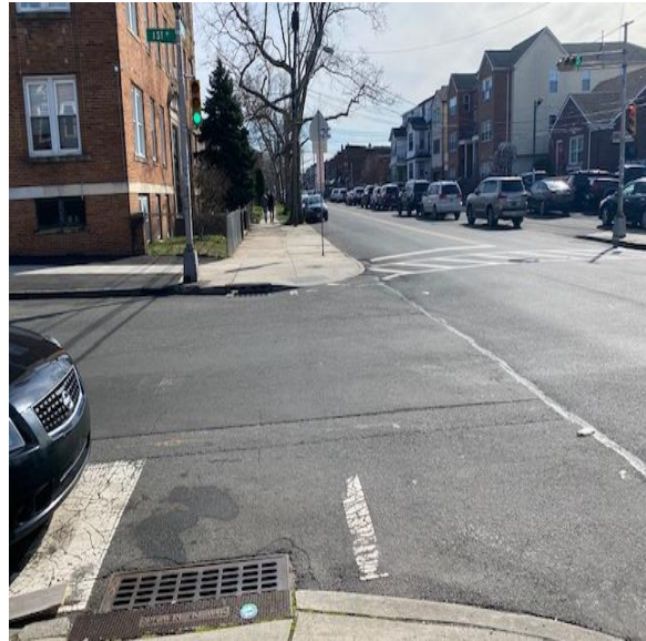
Completely faded crosswalk to cross 1st Ave. at Roseville Ave. needs to be repainted
