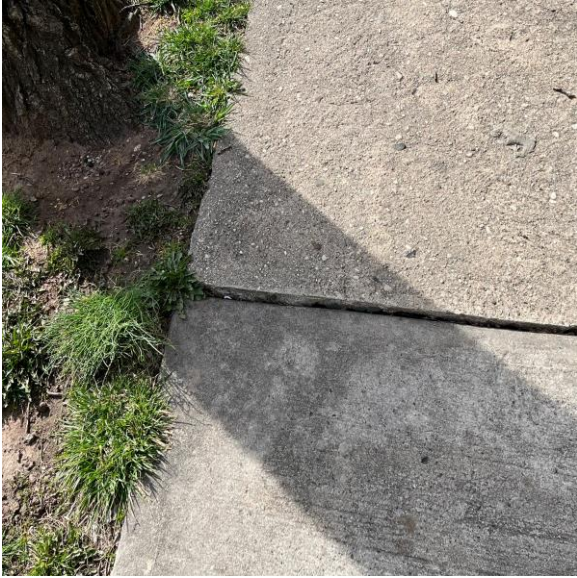
Sidewalk is tripping hazard due to tree roots 1st Ave.
