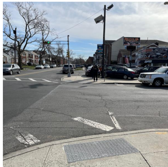
Need to repaint crosswalk, dome pad direction slightly off, no street lighting 1st Ave
