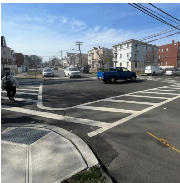
Dome pad directed toward middle of intersection, no street lighting Intersection of 2nd Ave. & N. 5th St.
