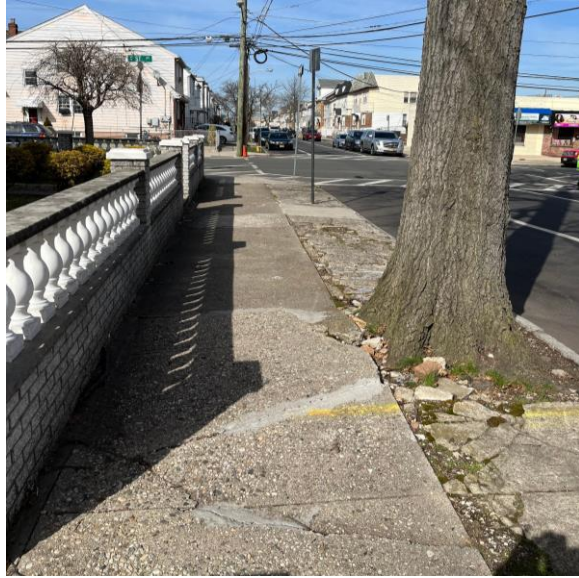
Sidewalk uneven from tree growth, and sidewalk to the right crumbling N. 11th St.
