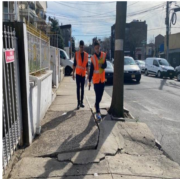
Tripping hazard on N. 7th btw. Bloomfield & Abington due to tree roots
