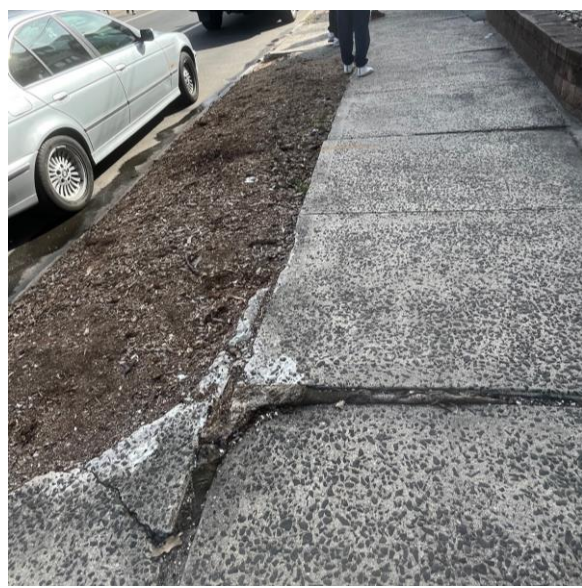
Sidewalk not level - trip hazard
