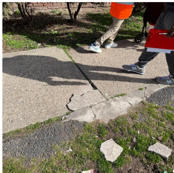
Sidewalk uneven and slightly cracked 481 Roseville Ave.
