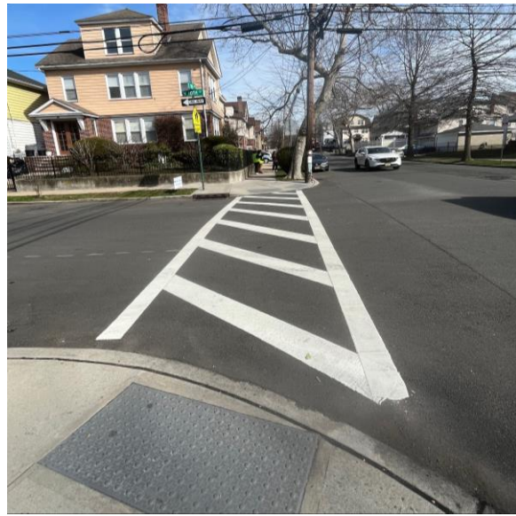
Dome pad direction slightly off Intersection of 2nd Ave. & N. 10th St.
