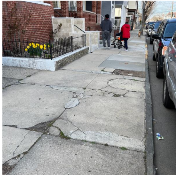
Sidewalk is cracked and tripping hazard 466 N. 6th St.
