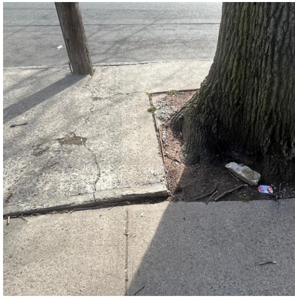
Sidewalk lifted and trip hazard from tree roots 1st Ave.
