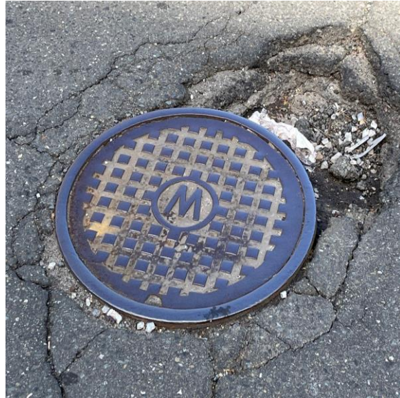
Big pothole in street next to manhole Intersection of 1st Ave. & N. 6th St
