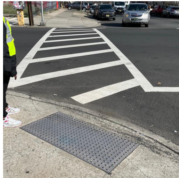
High visibility crosswalk, dome pad directed toward middle of intersection-not crosswalk 2nd Ave
