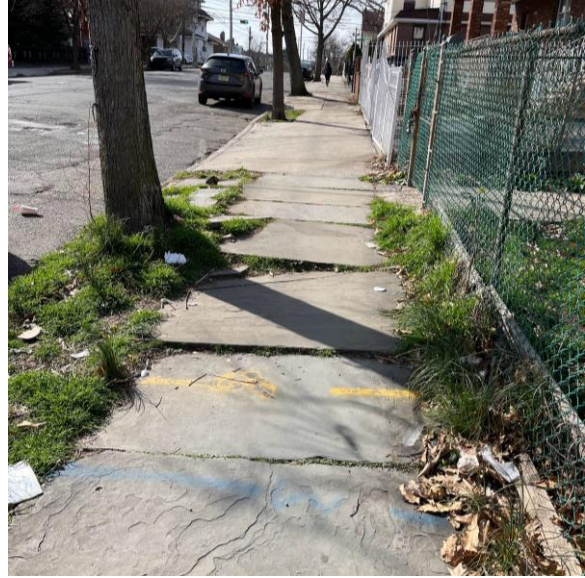
Sidewalk is a tripping hazard and strollers/wheelchairs may not have access Corner of 3rd Ave. & N. 7th St.
