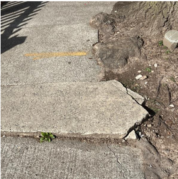
Sidewalk uneven from tree growth N. 11th St.
