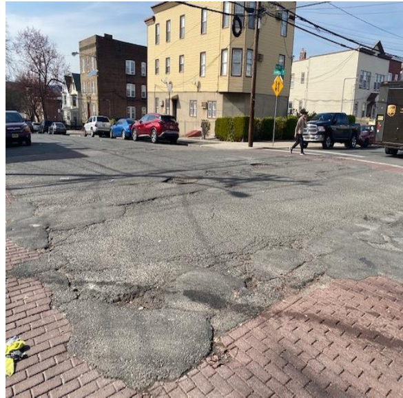
Damaged road and faded brick crosswalk borders w/ potholes at N. 7th & Berkeley
