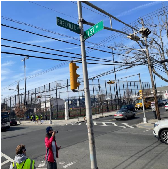
One light attached to the utility pole, Need stop bar for cars at 1st Ave. & Roseville
