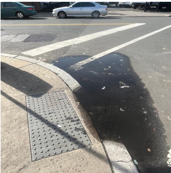
Poor drainage Intersection of 4th & Bloomfield
