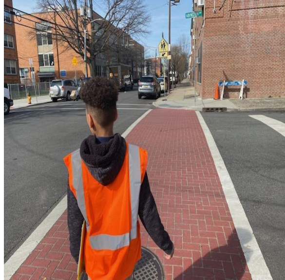
Low visibility brick crosswalk is a challenge for wheelchairs to roll over and may trip people in heels at N. 7th & Abington
