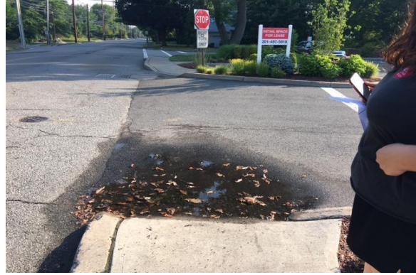
Fig. 2d. Curb ramp Lacks Dome Pad
