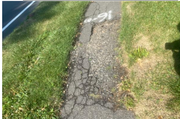
Fig. 4f. Broken sidewalk on Ridgewood
